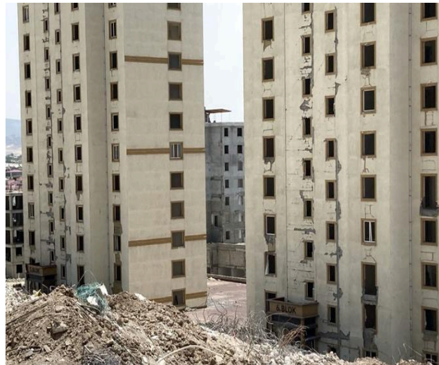
Figure 3 - Damaged tunnel-form buildings (Brzev et al., 2025)
