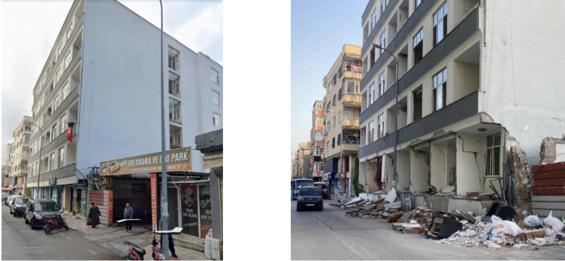
Figure 1 - Soft story collapse of a mixed residential/commercial RC building in the Hatay province (Brzev et al., 2025)
