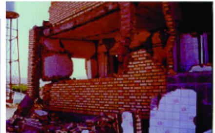
Figure 6B: Damage due to large opening, absence of masonry shear wall and short column behavior in concrete post (1990 Manjil earthquake)
