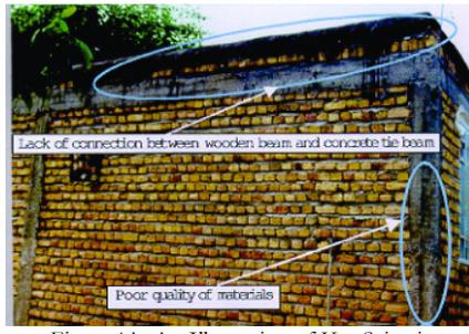
Figure 4A: An Illustration of Key Seismic Deficiencies: lack of Connection Between Wooden Beam and Concrete Tie Beam and Poor Quality of Materials
