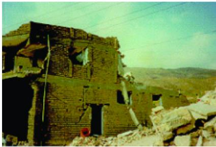
Figure 5: Damage caused by the absence of concrete posts (1990 Manjil earthquake)
