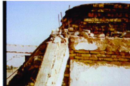
Figure 6D: Collapse due to heavy roof (1990 Manjil earthquake)
