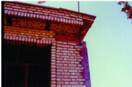
Figure 6C: Damage in the wall panel (1990 Manjil earthquake)
