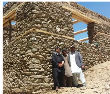
Fig. 4: Rubble stone wall with wooden logs (Photo source: solidarites.org)
