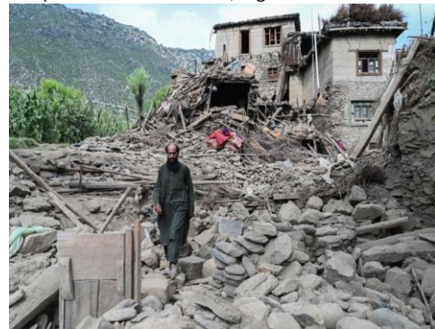
h) Destroyed houses in mountainous terrain after the August 2025 earthquake in eastern Afghanistan 6 .
