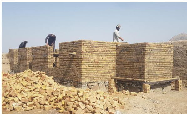
Fig. 3: Burned Brick wall with Stone masonry foundation (achro.org).
