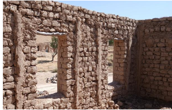
Fig. 2: Mud brick wall (achro.org)
