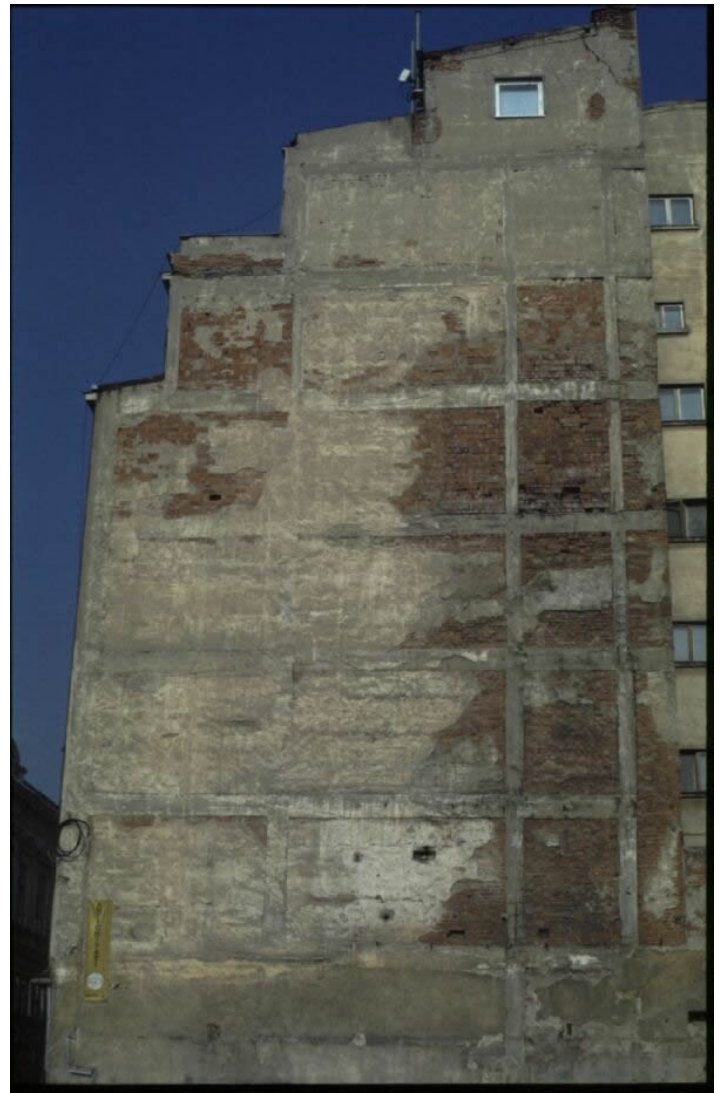
Side wall of a typical building (from Bostenaru(2004))
