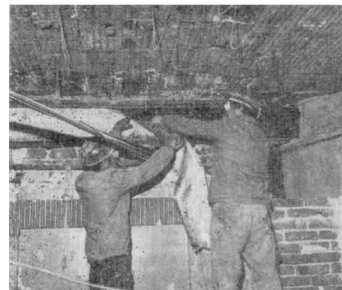
Application of the weaving over the resin layer
