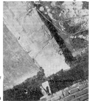
Beams plated with glas fibre weaving embeded in epoxy resin (black colour)
