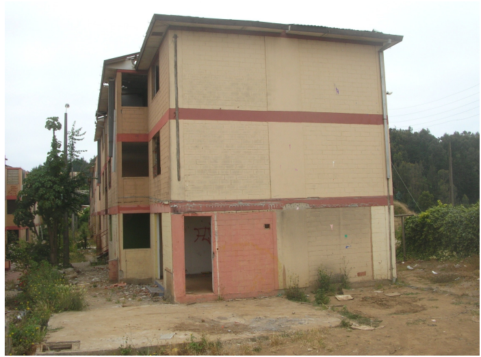
Opening of door in the first floor. Constitucion.
