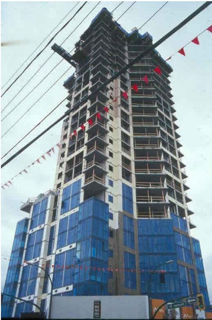
A Typical Building Under Construction
