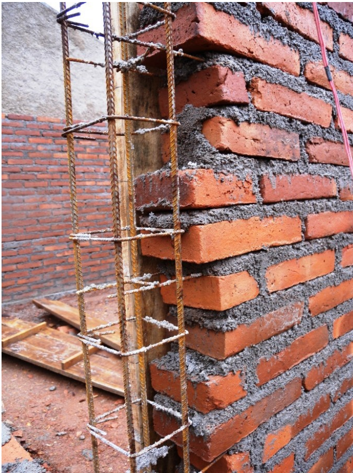
a toothed wall-to-tie-column interface
