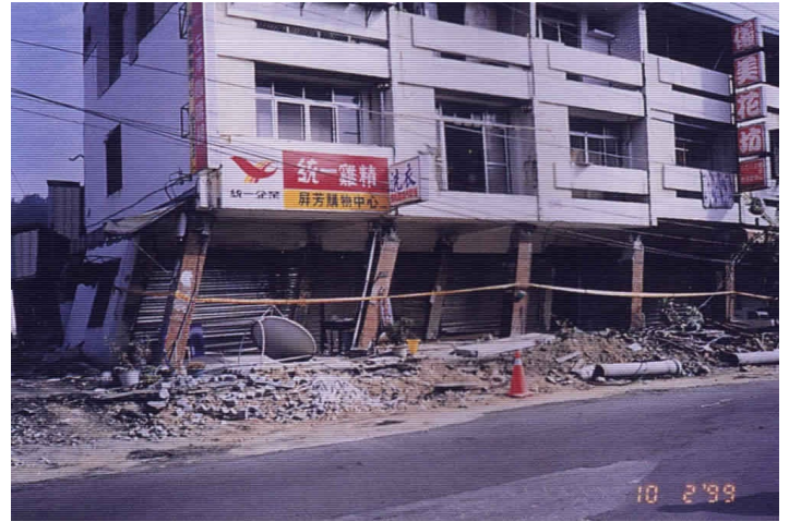
A Photograph Illustrating Typical Earthquake Damage
