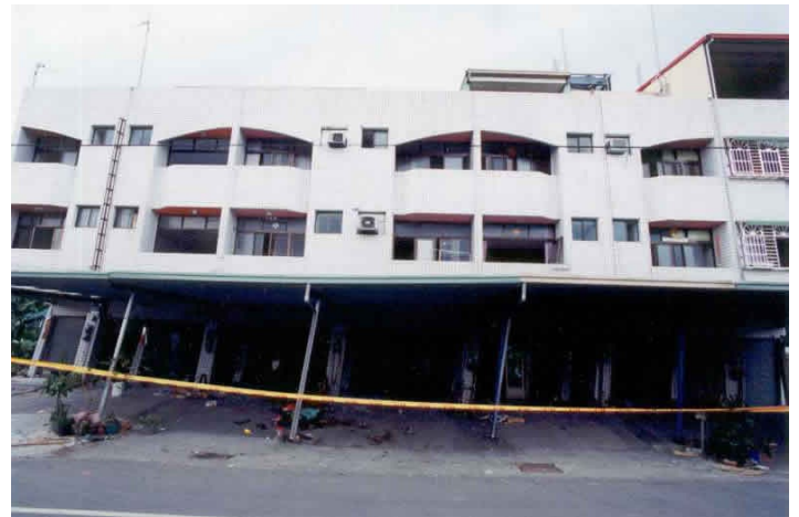
Earthquake Damage - Partial Collapse of a Three-story building in the 1999 Chi Chi Earthquake (Source: EERI 2001)
