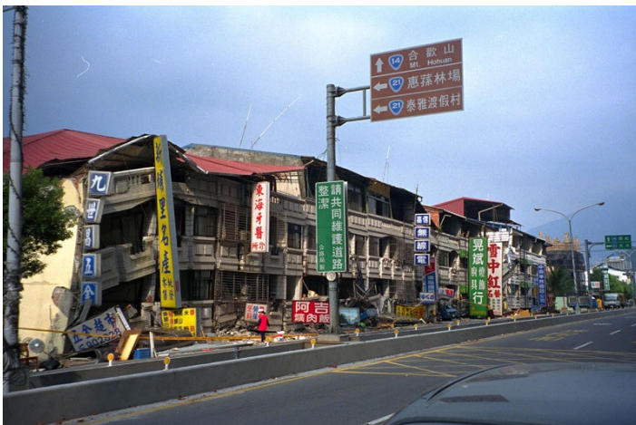
Earthquake Damage - Pancake Collapse of an Entire City Block in the 1999 Chi Chi earthquake (Source: EERI 2001)
