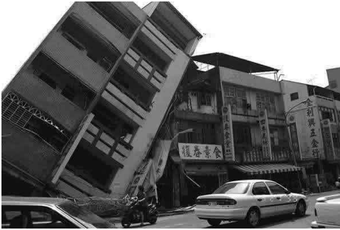
Collapse of a Concrete Frame Building in the 1999 Chi Chi Earthquake (Source: EERI 2001)
