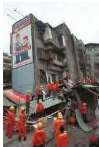
Earthquake Damage - Collapse of a 5-story building in the March 31, 2002 Taipei earthquake
