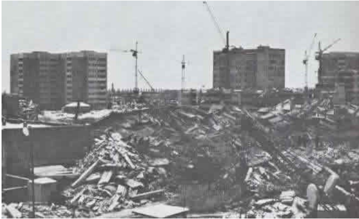
Earthquake Damage - Large Panel Buildings Remained Undamaged in the 1988 Spitak (Armenia) Earthquake (Source: EERI Armenia Earthquake Reconnaissance Report)
