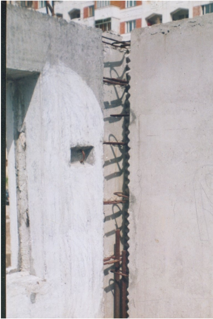
Critical Structural Details- Vertical Wall Panel Joint
