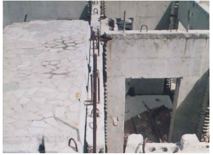
Critical Structural Details - Erection of Floor Panels
