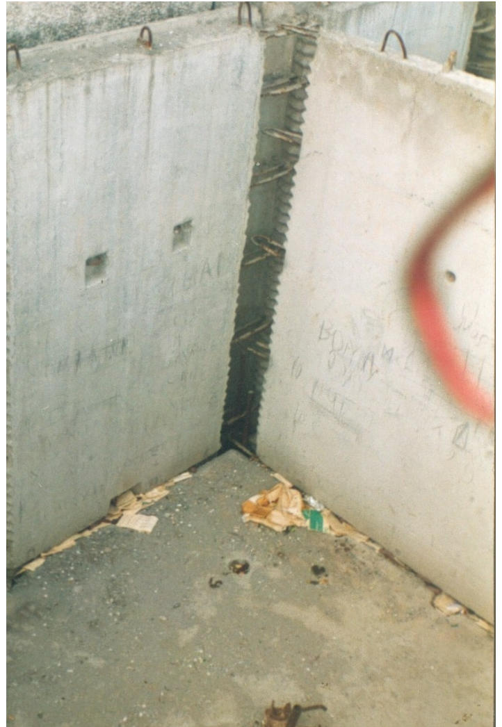
Critical Structural Details- Vertical Wall Panel Joint
