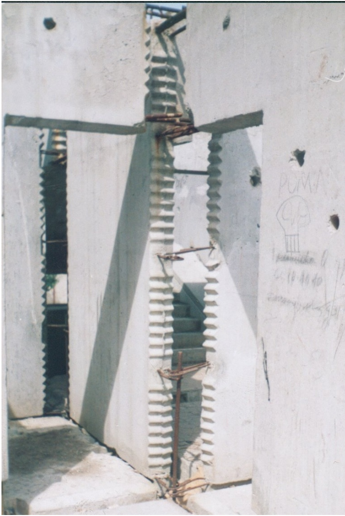
Critical Structural Details- Serrated Wall Surfaces
