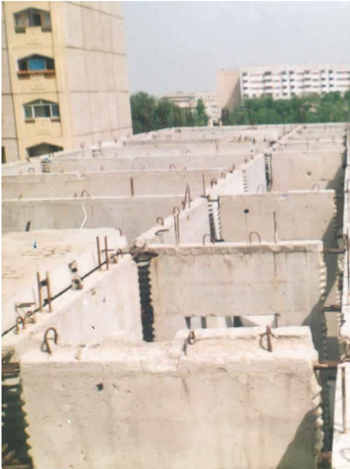
Critical Structural Details- Wall and Floor Panels
