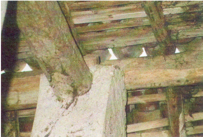
Critical Structural Detail - Roof Beam Support
