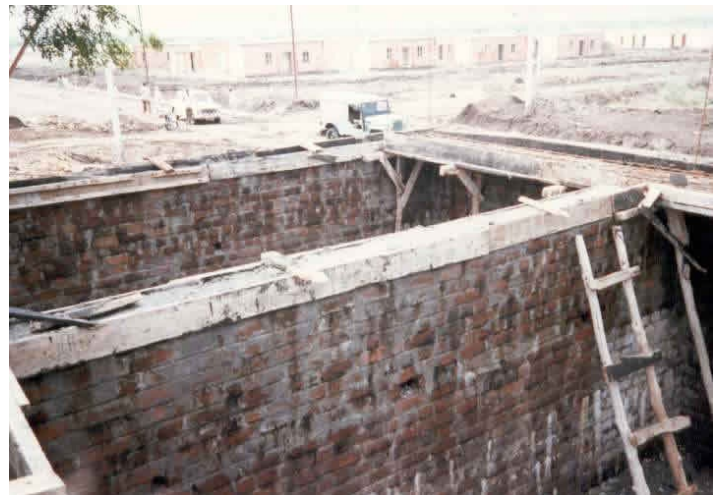
Construction of RC Lintel Band - Pouring of Concrete Completed
