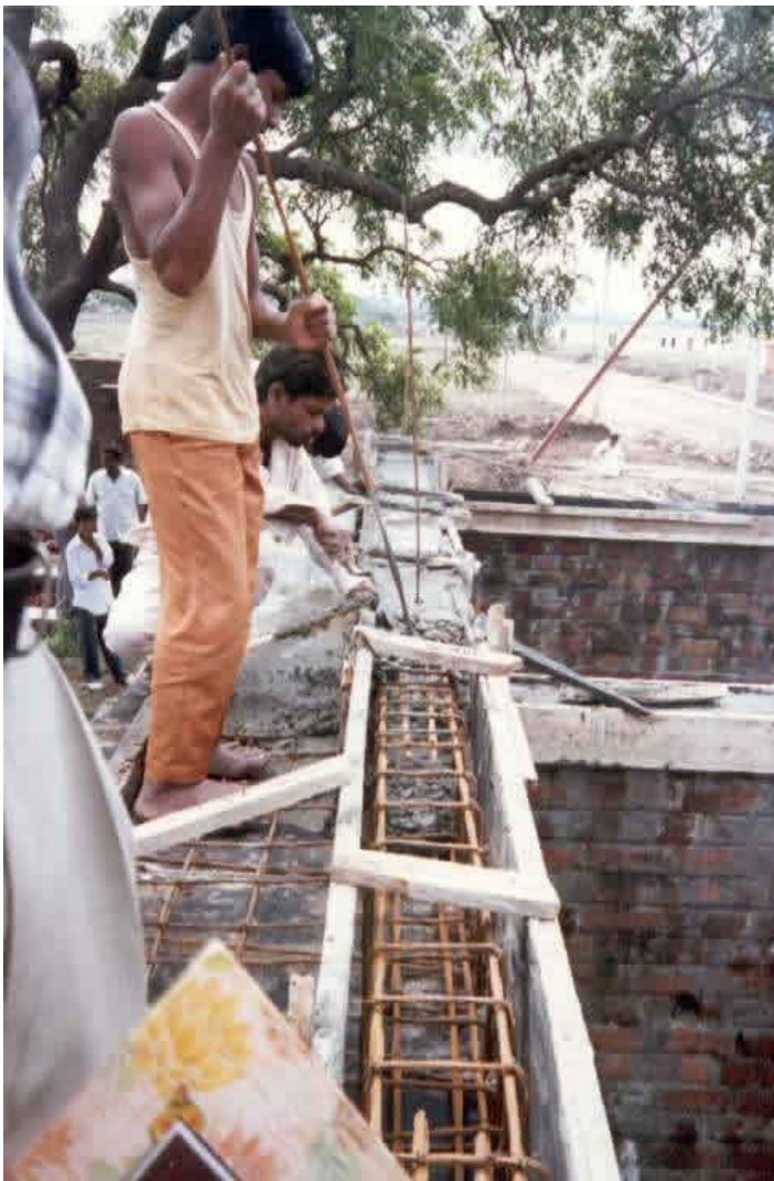
Construction of RC Lintel Band
