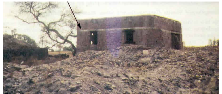
Key Seismic Resilient Features - RC Lintel Band and Good Quality Construction; note example of a building that sustained the effects of the 1993 Killari earthquake (M6.4) without damage although located very close to the epicentre
