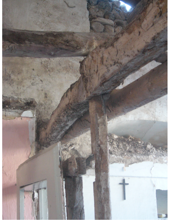
Figure 9. Timber frame supporting the vault
