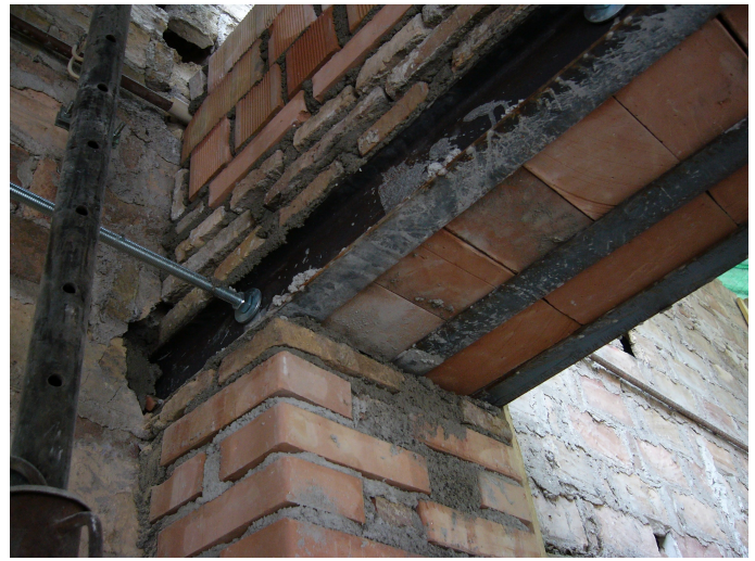
Figure 20. Replacement of the old brick lintel with a new reinforced one
