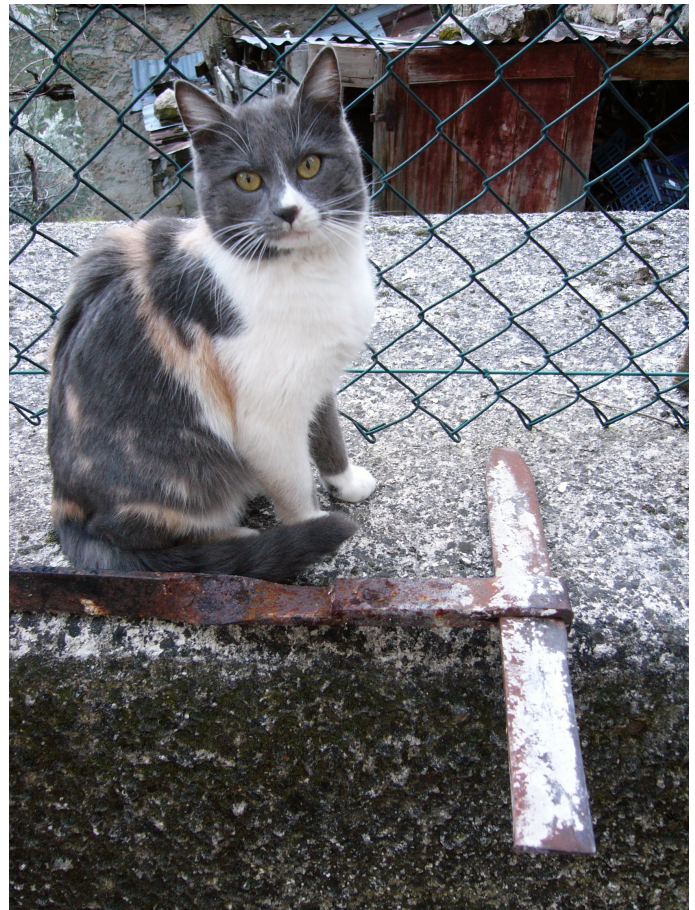
Figure 11. Old metallic tie placed to achieve the box-behaviour of the structure
