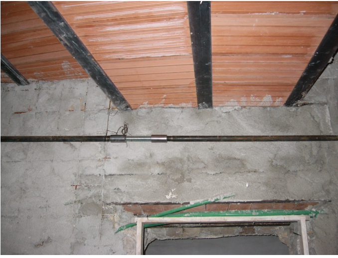
Figure 15. Placement of metallic ties to achieve the box-behaviour of the structure
