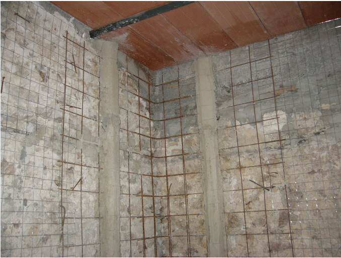
Figure 17. Construction of concrete jackets on both faces of the walls
