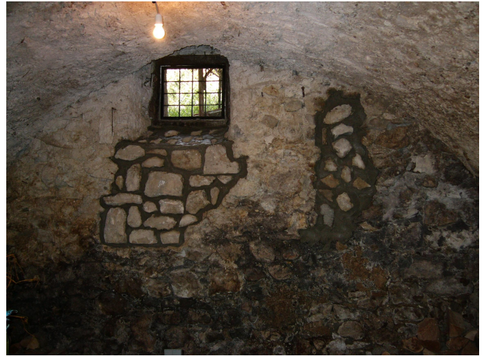
Figure 18. Scuci - cuci patching
