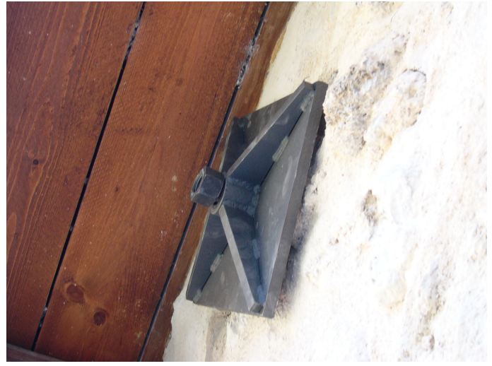
Figure 16. Placement of metallic ties to achieve the box-behaviour of the structure
