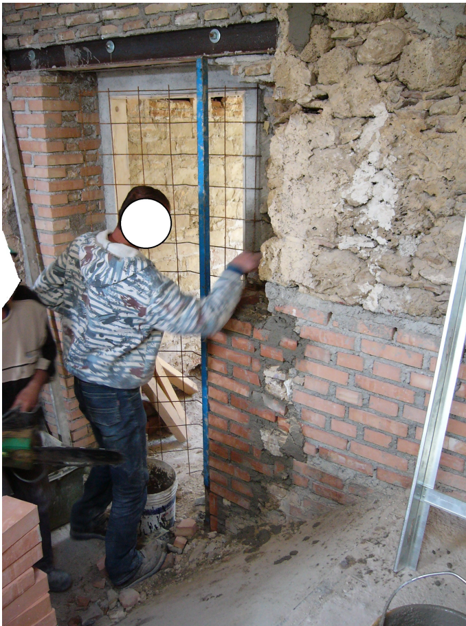
Figure 19. Reinforcement of the jamb and new lintel
