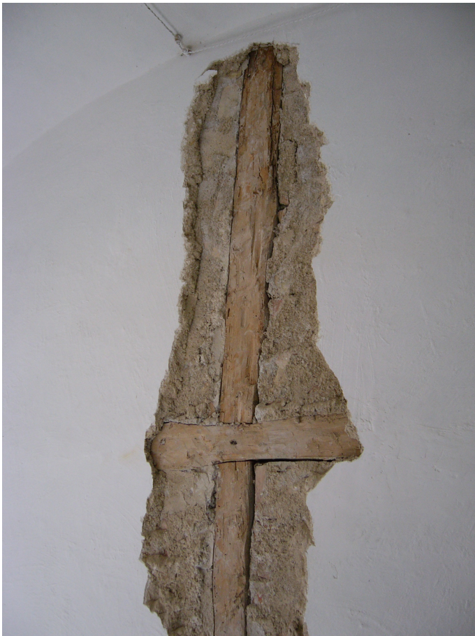
Figure 10. Inner structure of a wall underneath the plaster
