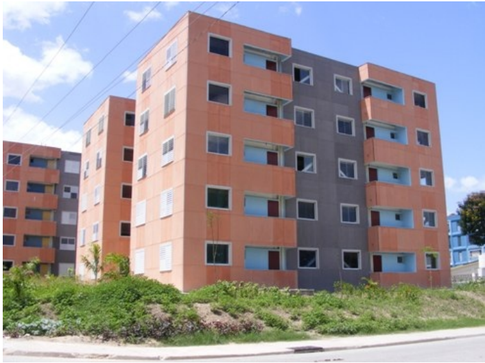
Figure 3. RC shear walls
