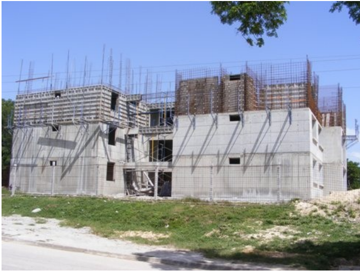
Figure 2. Construction of FORSA building
