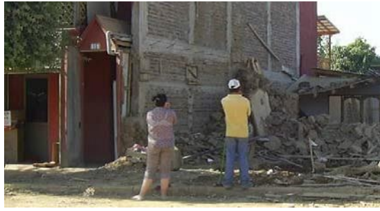
Figure 12. A two story confined masonry house in Curepto after 2010 earthquake which remained virtually undamaged, while the adjacent adobe house collapsed (Meli et al., 2011).
