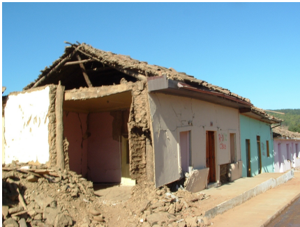
Figure 11.b Collapse of adobe houses in 2010 Maule earthquake in the city of Curepto
