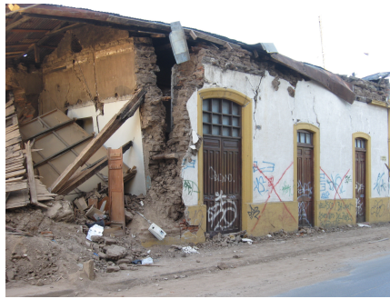
Figure 11.a Collapse of adobe houses in 2010 Maule earthquake in the city of Talca
