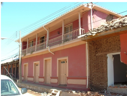
Figure 1.b Typical adobe houses in the city of Curepto, central Chile
