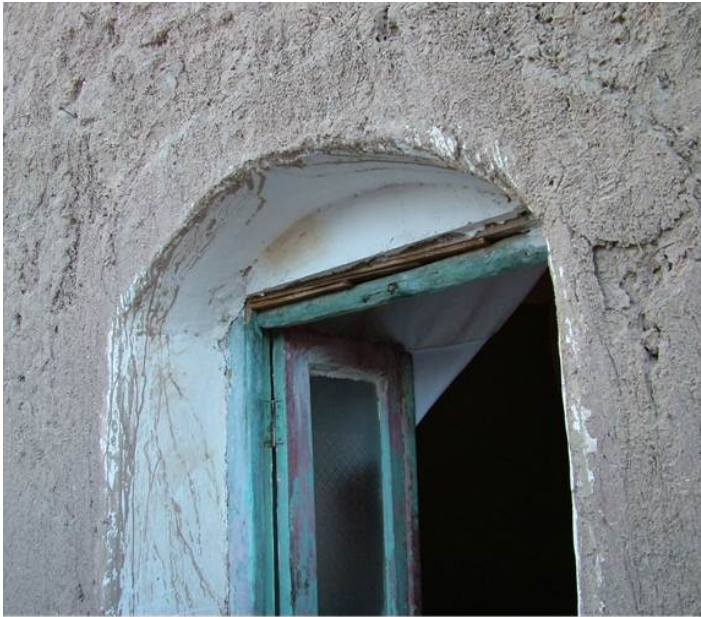
Figure 6. Different types of opening: (a) arched without lintel
