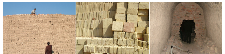
Figure 9. Construction of sun-dried, baked square and rectangular adobe blocks: (b) Kerman province
