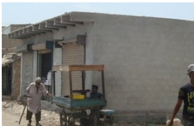
Block masonry with concrete girder roof and concrete tiles.
