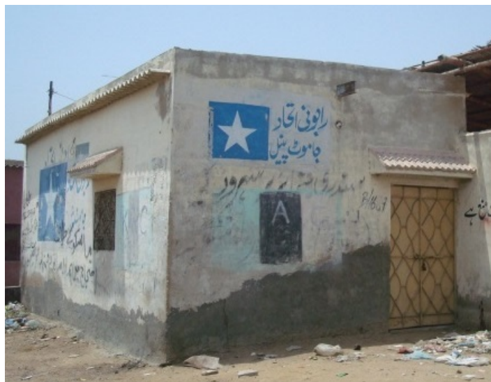
Block masonry with CGI sheet roof held down by a plastered parapet of blocks.
