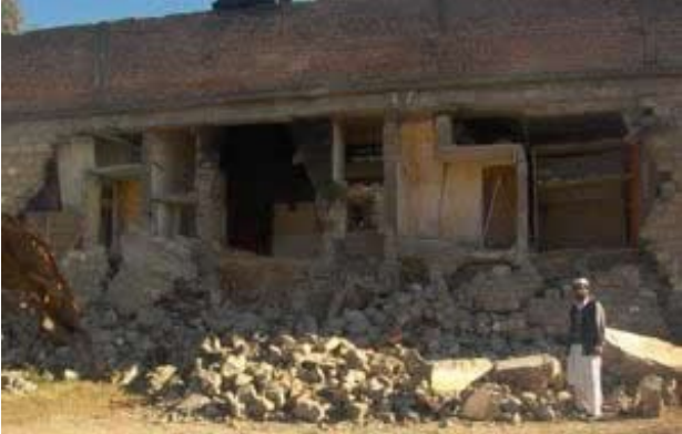
Out of plane flexural failure of load bearing wall constructed with block masonry in Kashmir Earthquake of 2005 [4].
