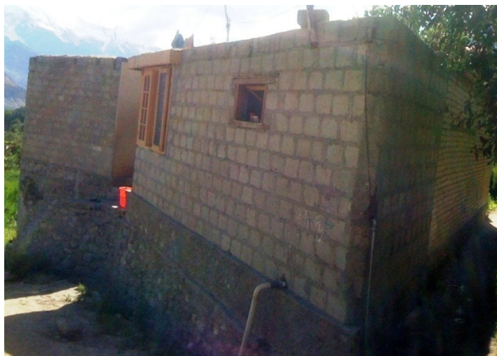
Stone plinth and foundation underneath block masonry.
