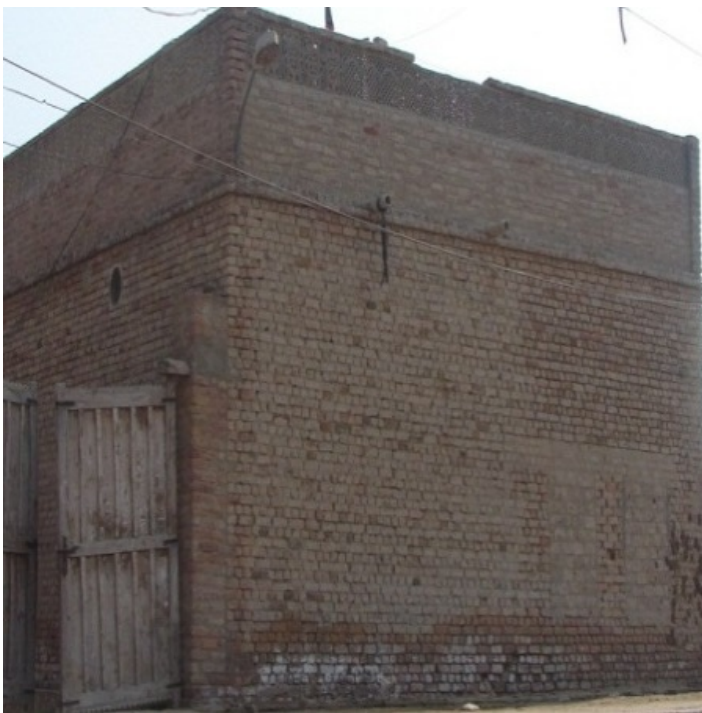
Brick masonry walls.
