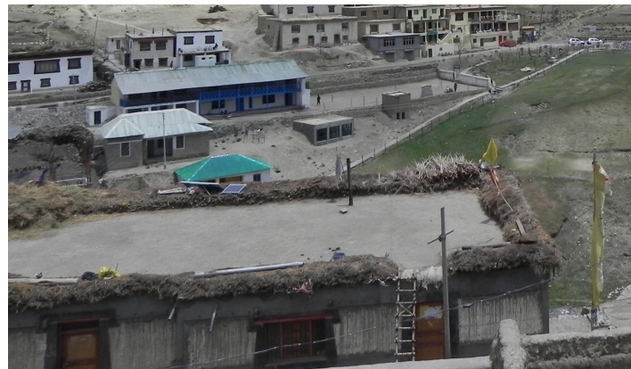
Parapet over a Spitian house terrace.
