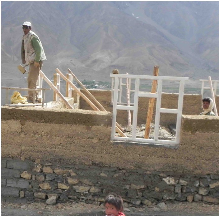
Walls with already placed window frames.
