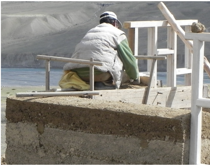
Wooden formwork to lay courses of mud.
