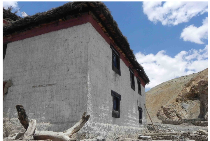
Bushes projecting outwards, hence forming a type of sunshade/roof projection.
