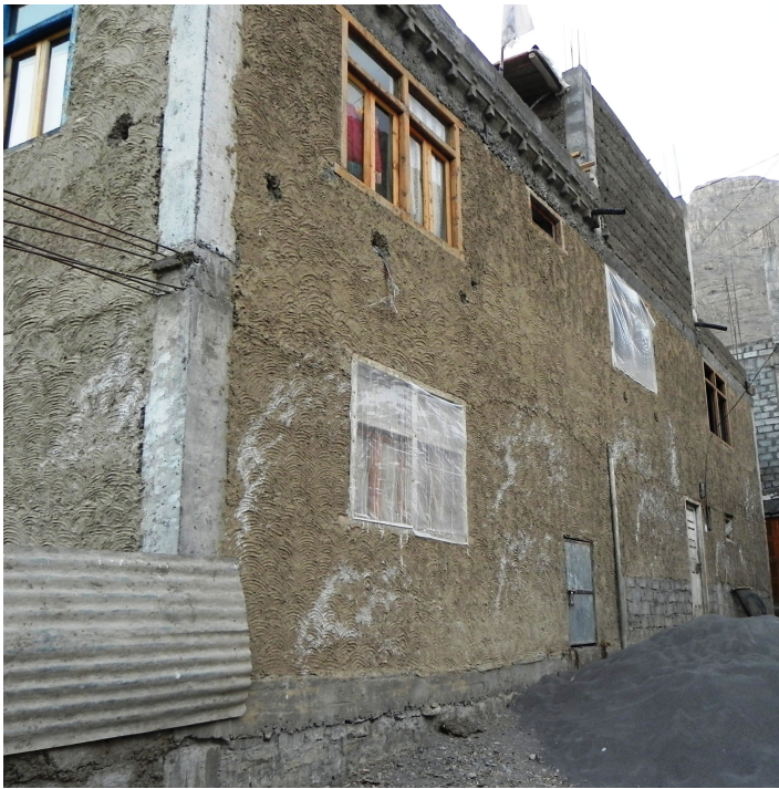
RC framed structure with mud walls infill and mud roof.
