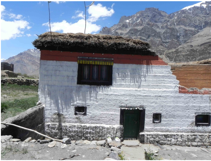
Lower portion of the wall made up of field stones. The front door is arranged at ground floor level without any plinth.
