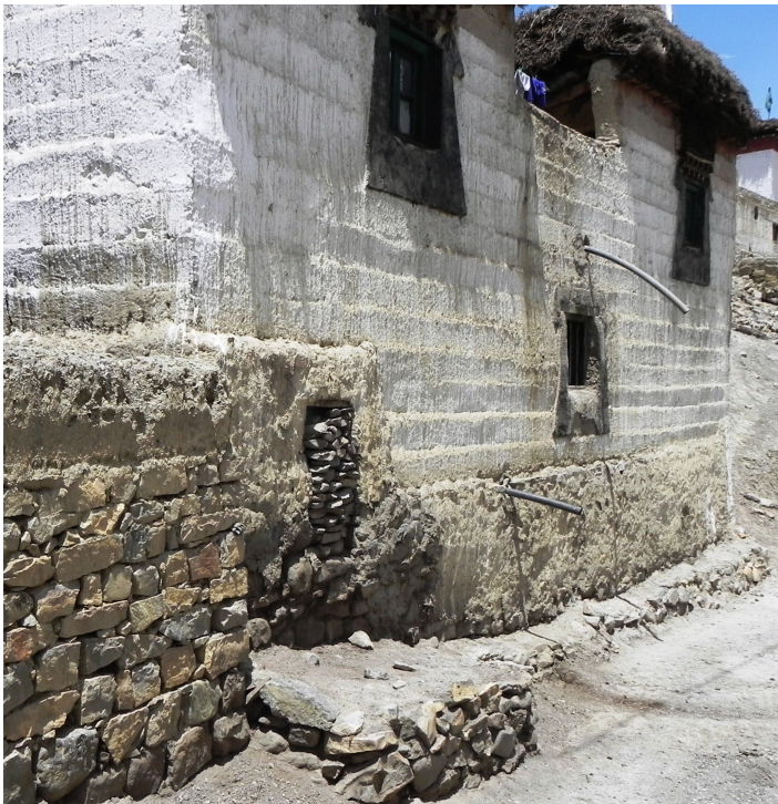
Over-ground septic tank's opening can be seen at ground floor level.
