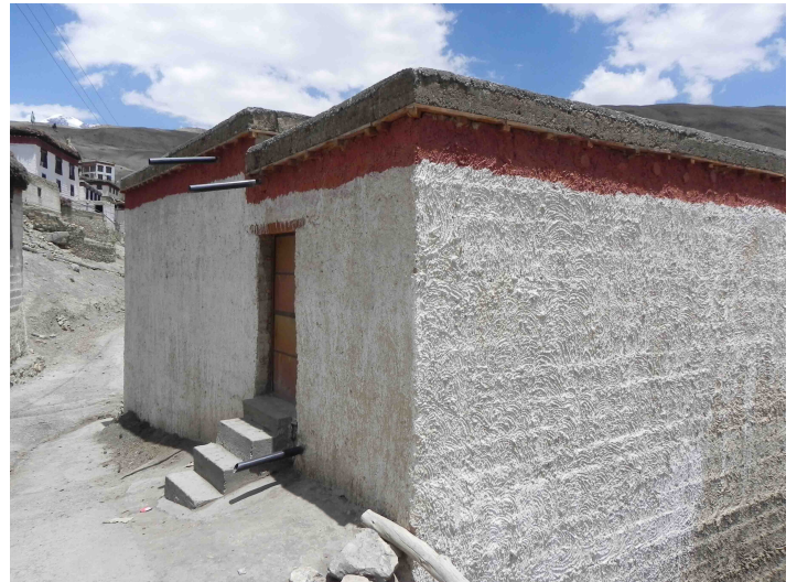
Patterns made to the outer walls with mud slurry for finishing.
