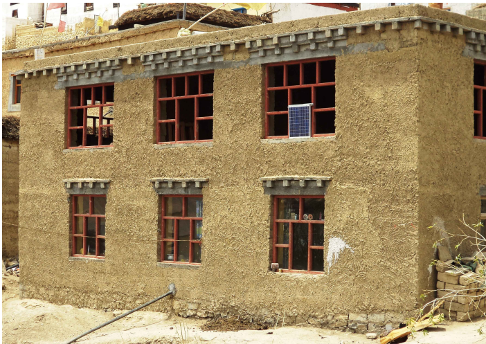
Precast RC lintels in a new construction.
