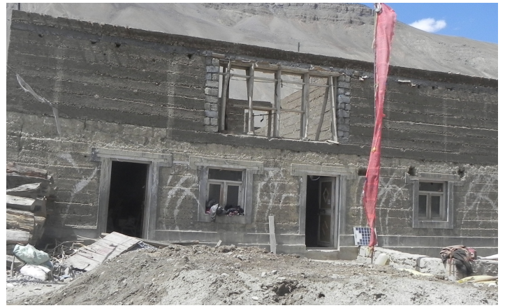
Marks can be seen on the wall of the upper floor where windows have to be cut. Lintel beams have already been provided during the wall construction process.
