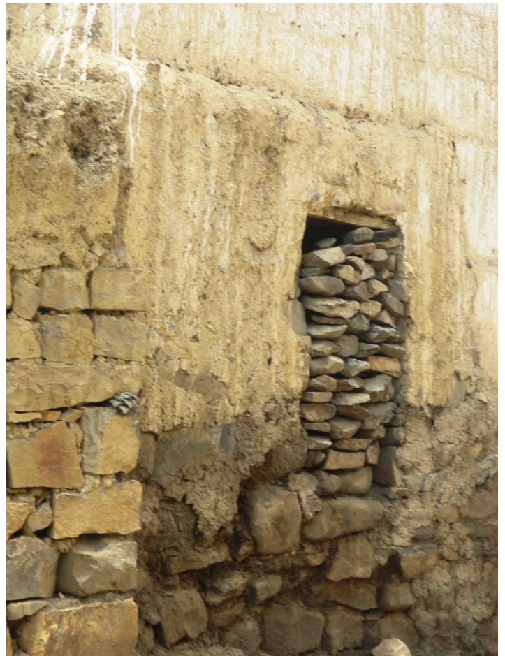
Septic tank's opening closed with dry stone packing.
