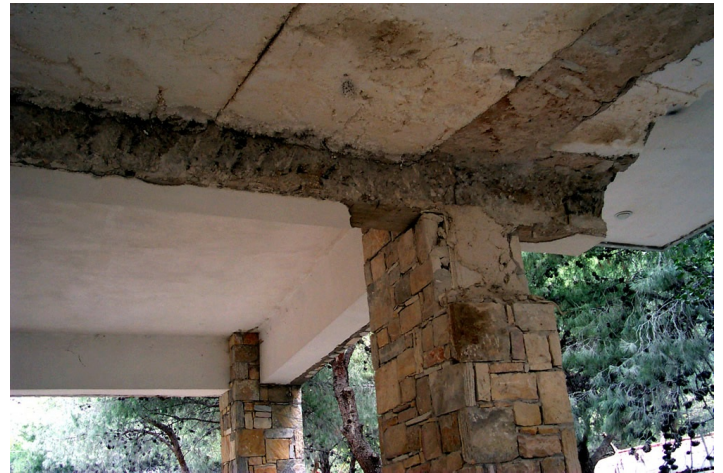
Critical Structural Elements: Column-Floor Slab Connection (1980 Structure)
