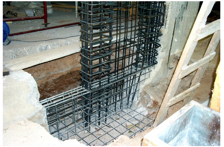
Seismic Strengthening of the Footing
