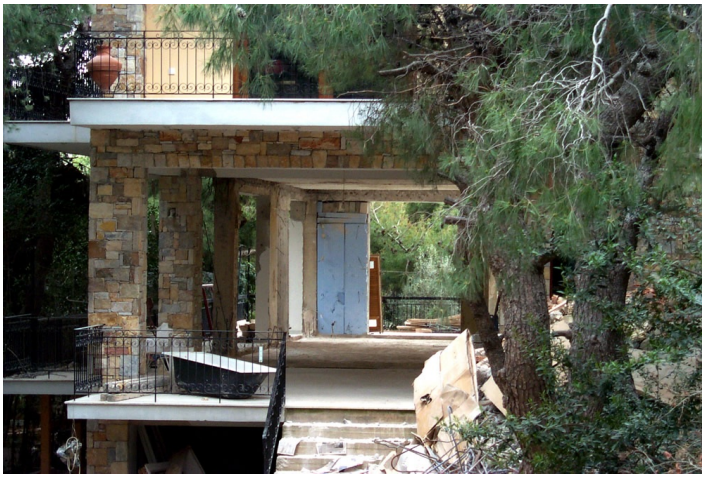
Demolition of the Damaged Infill Walls at the Ground Floor Level
