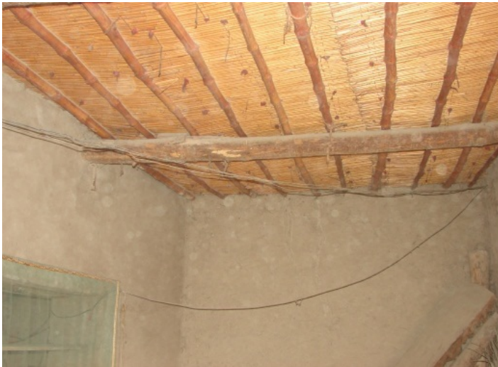
Adobe house roof - interior. Timber planks with bamboo stalks supporting wooden chick.
