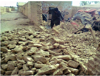
Typical damage caused by the Dalbandin earthquake in 2011.
