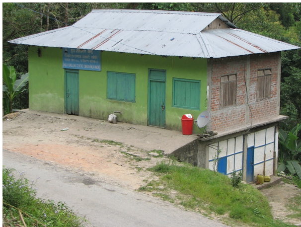
A vulnerable modification to the Ikra-type housing in Sikkim: heavy masonry infill walls above and light-weight Ikra walls below.
