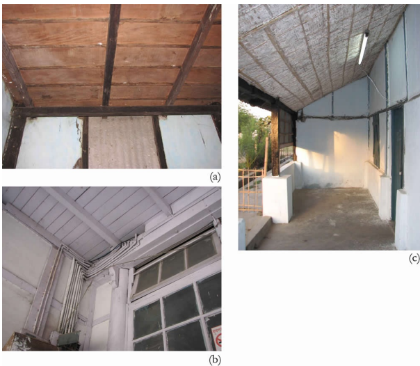
Commonly used roofing system: (a) CGI sheets, and (b) Ikra reed.
