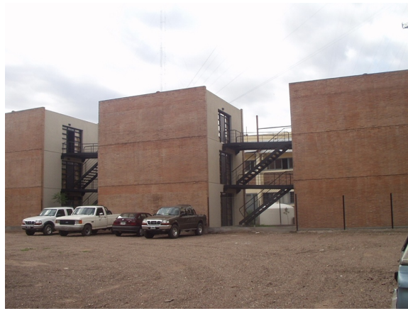
View of confined masonry buildings (South)
