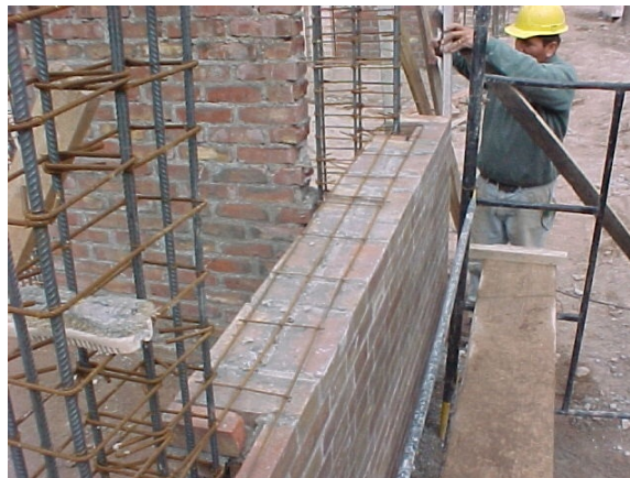
Construction of Reinforced Masonry
