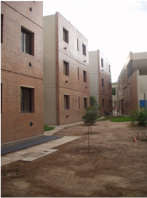
View of confined masonry buildings (North)
