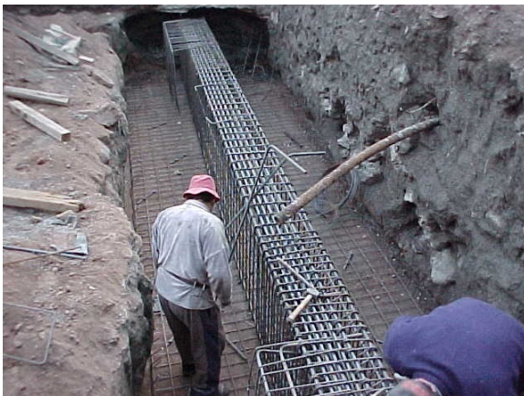
Construction of Reinforcement of Footings of BS1 Building (B1x and B2X)
