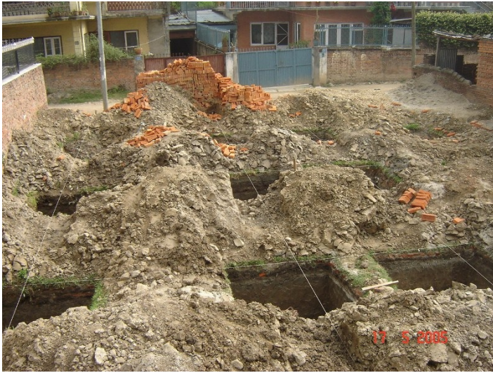
Pits for isolated footings
