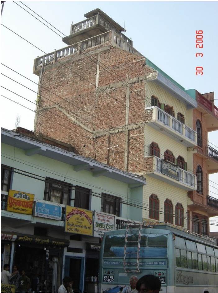
Column starting from 5th storey
