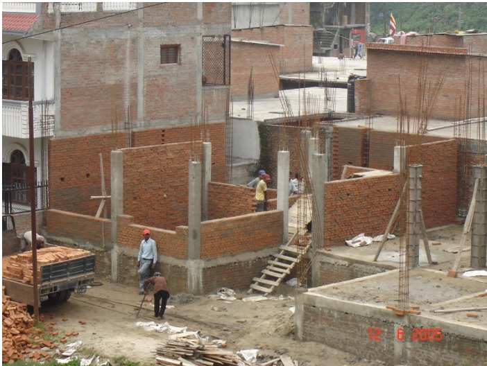
Infill wall under construction
