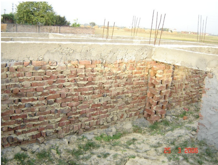
Toe wall below tie beam in mud mortar
