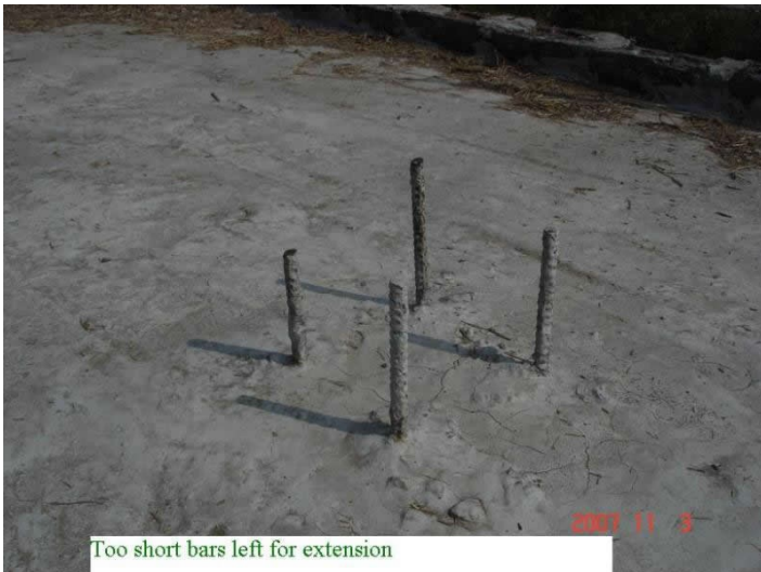
Column reinforcement is far too short for the continuity of the column
