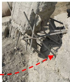
Deficient lap length, and very poor lap location leading to partial collapse of the building
