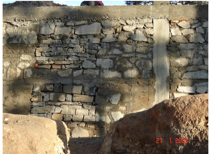
Infill wall in stone masonry
