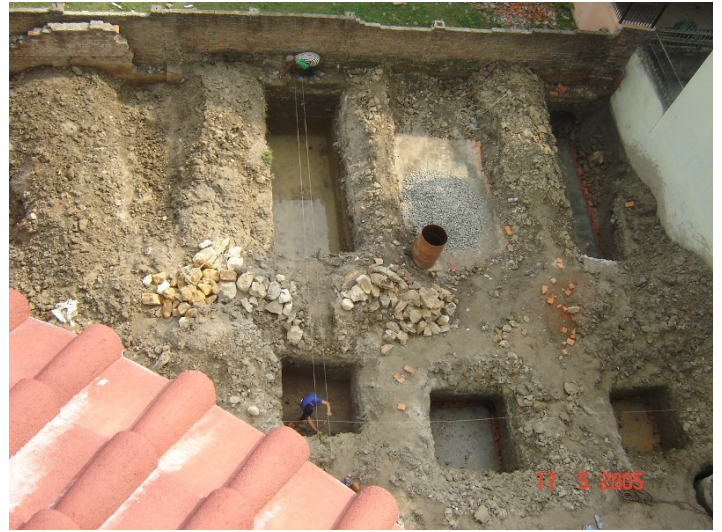
Pits for combined foundation
