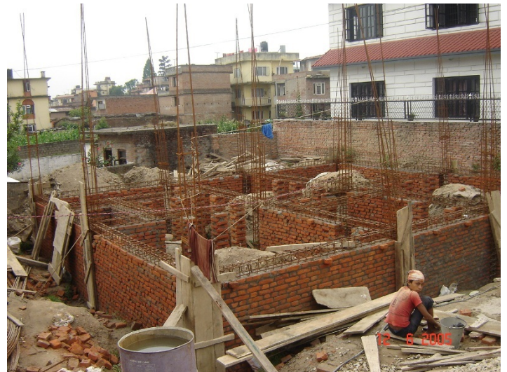
Plinth/ tie beam construction
