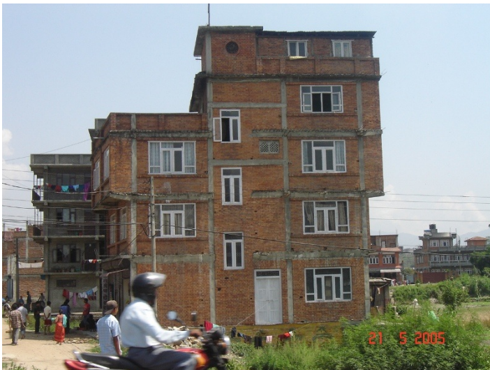
Missing beams
