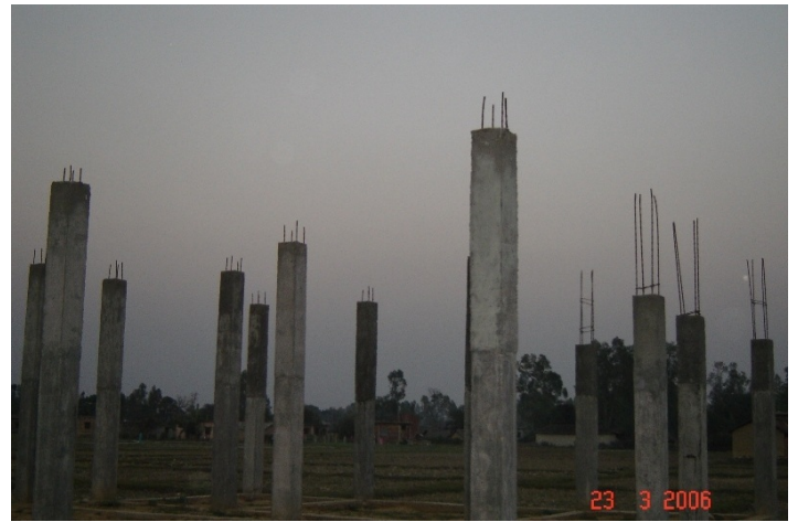
Column reinforcement left for splicing of upper story column reinforcement
