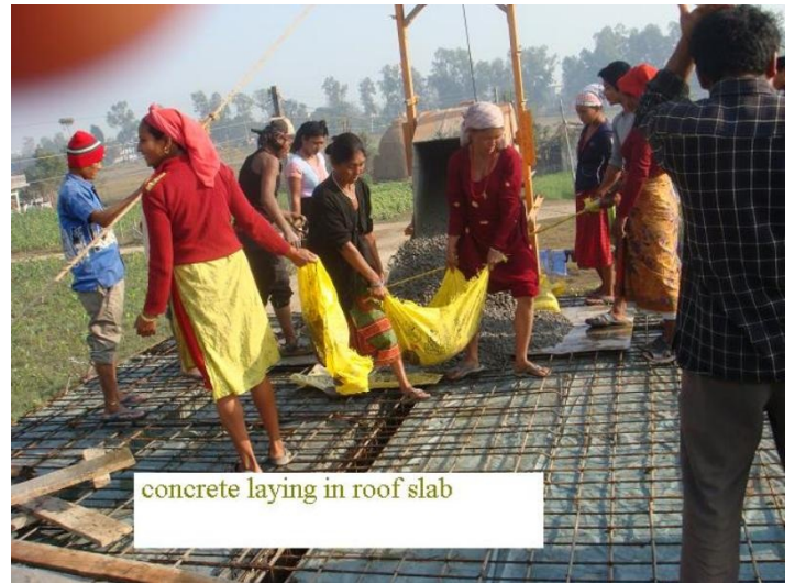
Construction of floor slab
