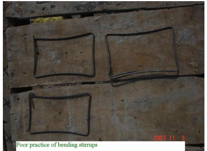
Defective stirrups due to 90 degree bends
