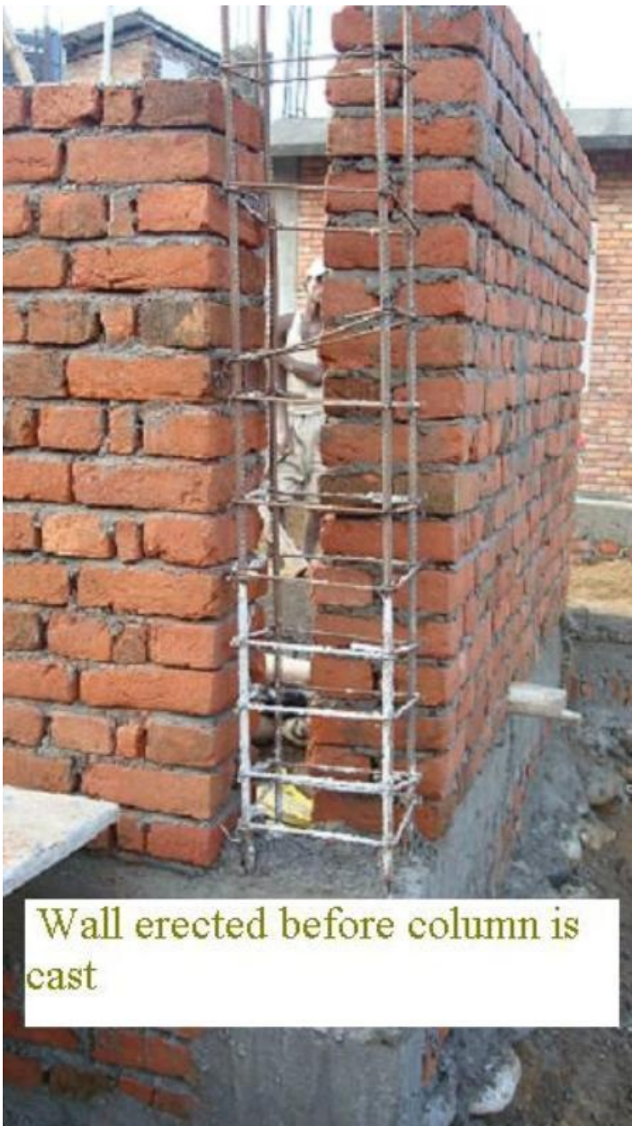
Infill wall erected before concreting column
