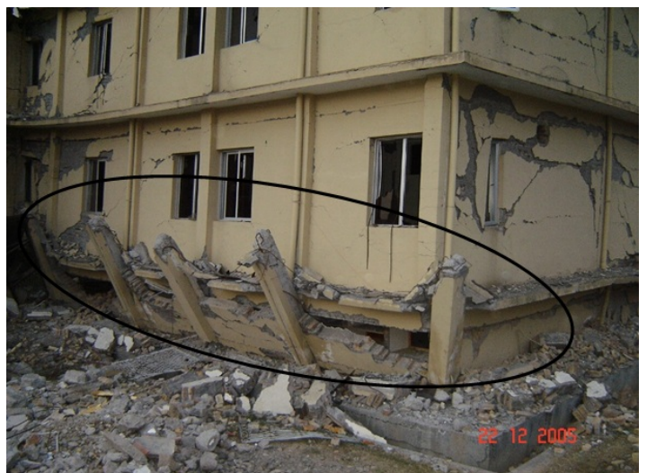
Failure of column bar splicing
