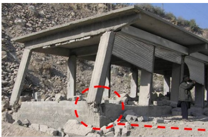
Deficient lap length, and very poor lap location leading to partial collapse of the building
