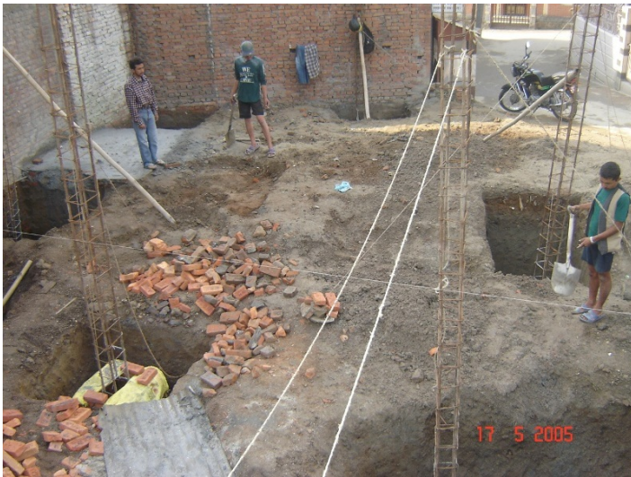
Isolated footings under construction
