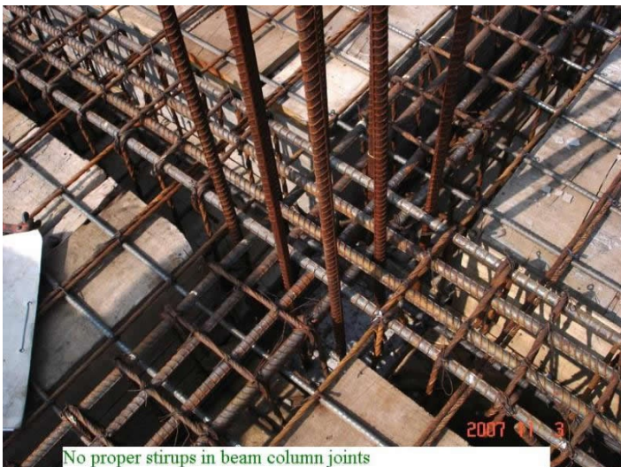
Column reinforcement is far too short for the continuity of the column
