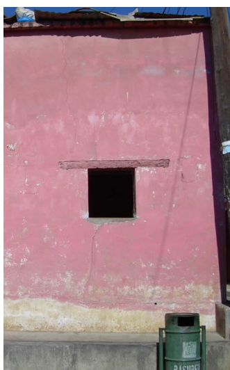
Window lintels consisting of wooden trusses.
