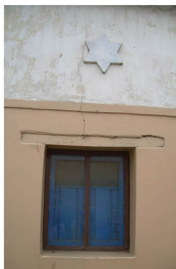
Window lintels consisting of wooden trusses.
