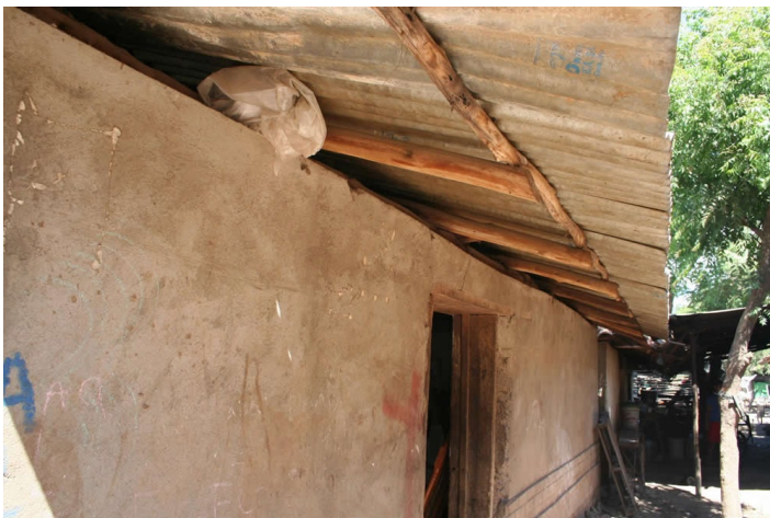
Timber roof framing and plastered wall.
