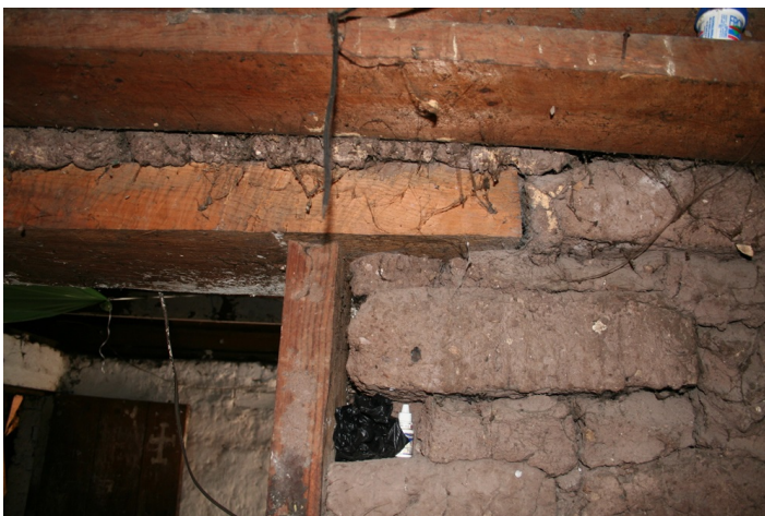
Lintel and wall connection.
