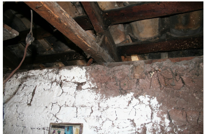
Roof framing and wall connection.
