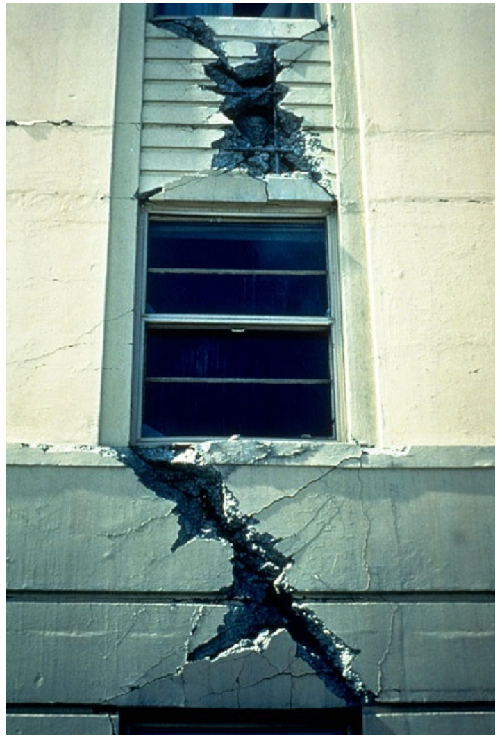
Close-up of characteristic X-shaped cracks and failure of coupling girders or short spandrel girders in the L street apartment building, Anchorage, Alaska. These girders were not properly designed for the shear demands. [10]
