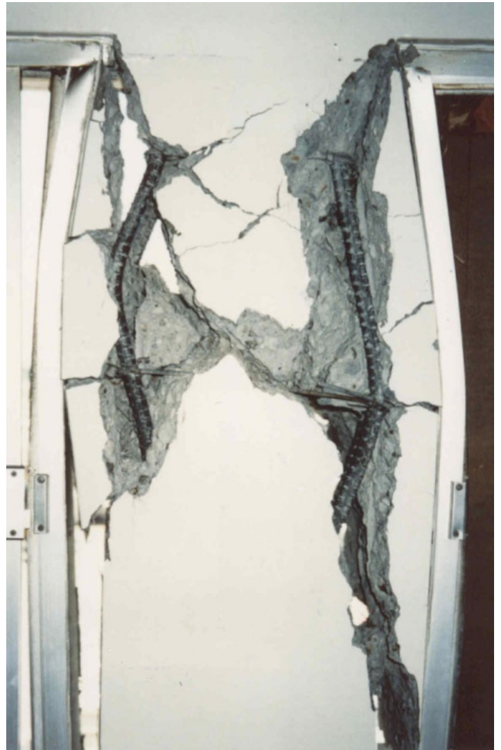
Damage to the Holiday Inn, Van Nuys primarily consisted of shear failure of the columns and subsequent buckling of column vertical reinforcing between the ties where added confinement provided by the concrete cover was no longer available,
