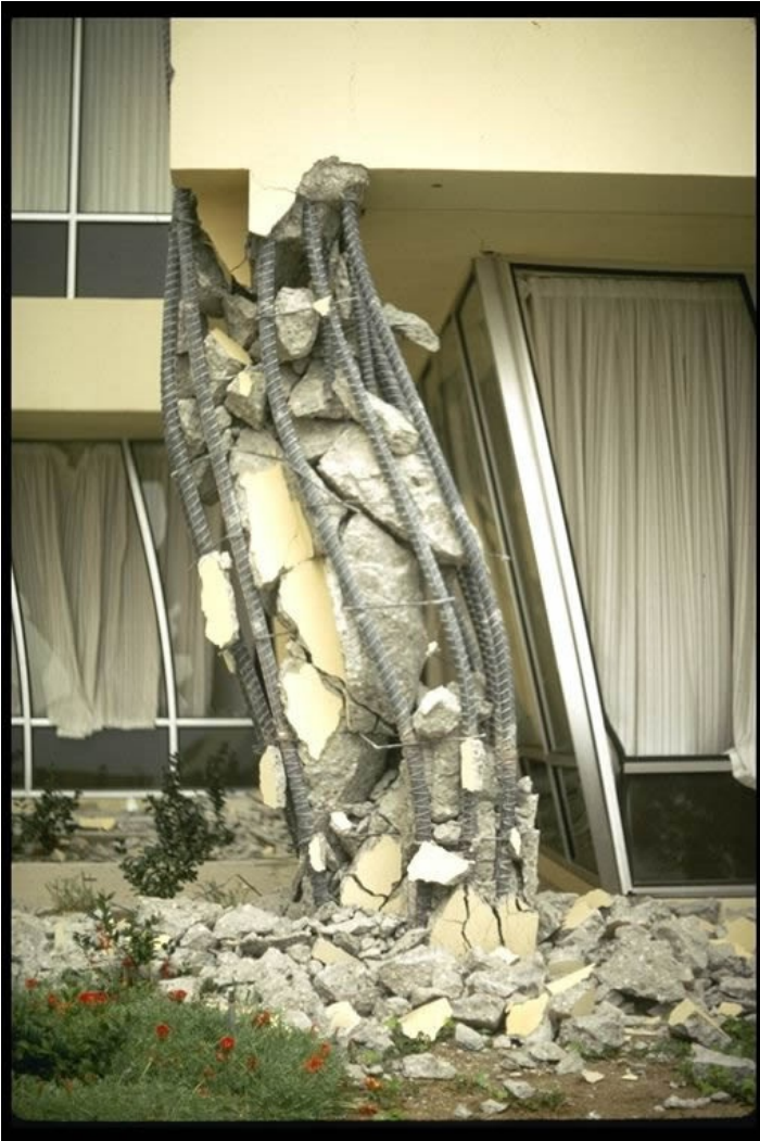
Example of damage to the corner columns at Olive View Hospital which was the result of poor seismic detailing. [9]
