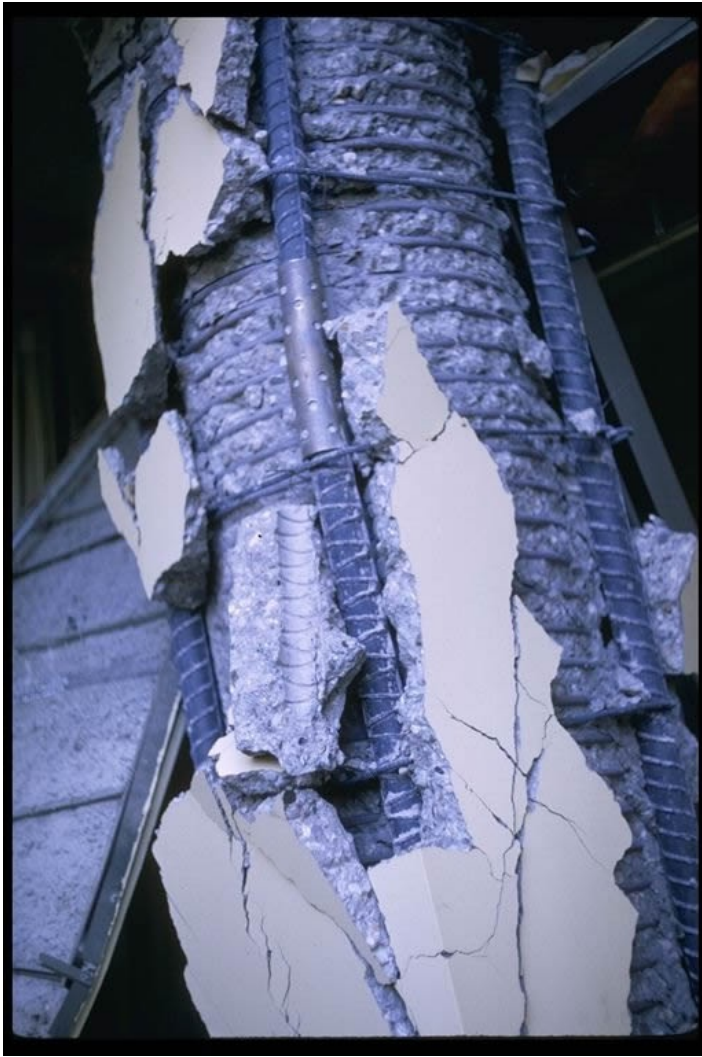
Detailed view of column with spiral confinement steel. The spiral confinement steel helped keep the concrete core intact. The longitudinal reinforcement is tied on the exterior of the spiral; this detail leaves the longitudinal steel vulnerable.
