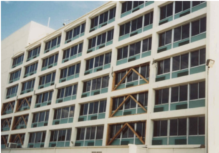
View of Holiday Inn, Van Nuys, CA with damage from the 1994 Northridge earthquake. The lateral system consists of reinforced concrete perimeter moment frames.
