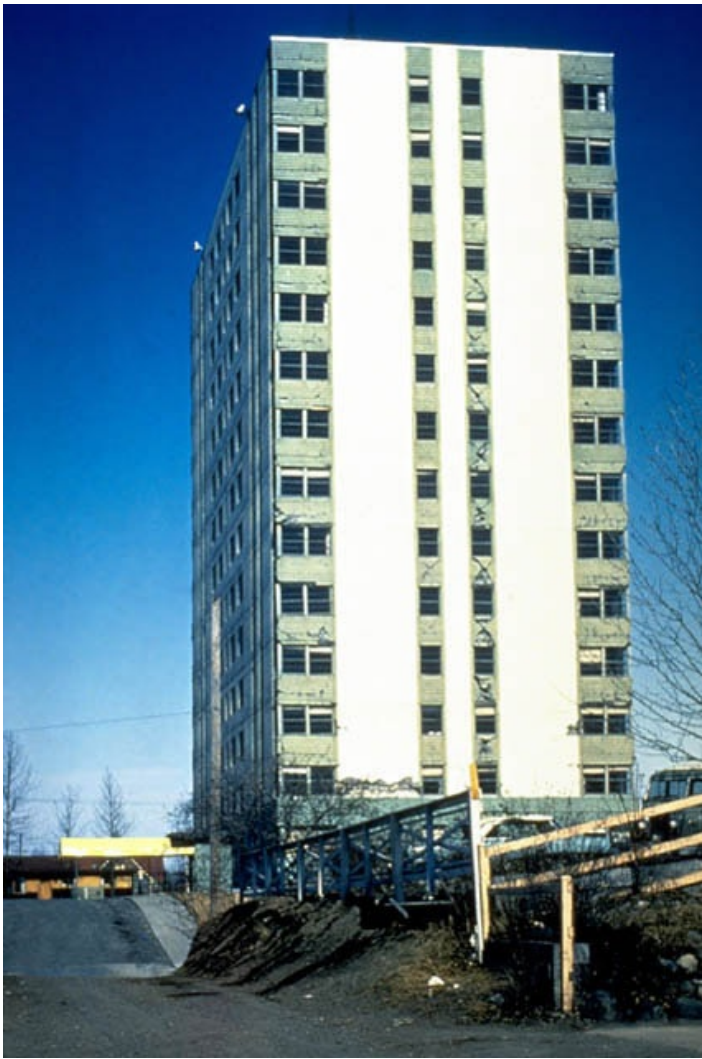
Overall view of the 1200 L Street Apartment building, Anchorage, Alaska after damage from the 1964 earthquake. This 14-story reinforced concrete structure has a basic lateral-resisting structural system and a series of slender walls
