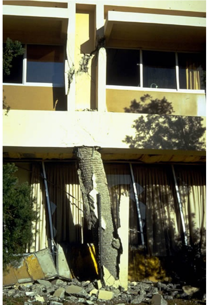
Detail view of the behavior of one of the first and second story columns in the Olive View Medical Treatment and Care Unit during the 1971 San Fernando Earthquake. Note the large permanent distortion of the first story column.
