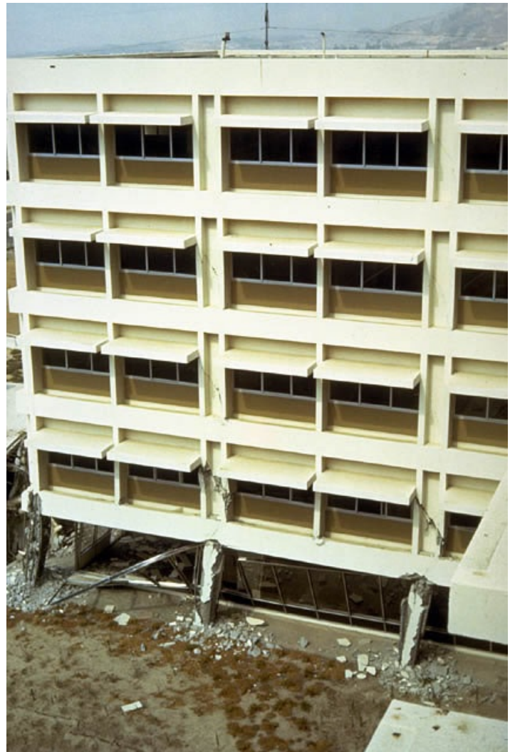
Olive View Hospital, Medical Treatment and Care Unit, 1971 San Fernando earthquake. View of the end of one of the four wings of this 5-story reinforced concrete building after the earthquake.
