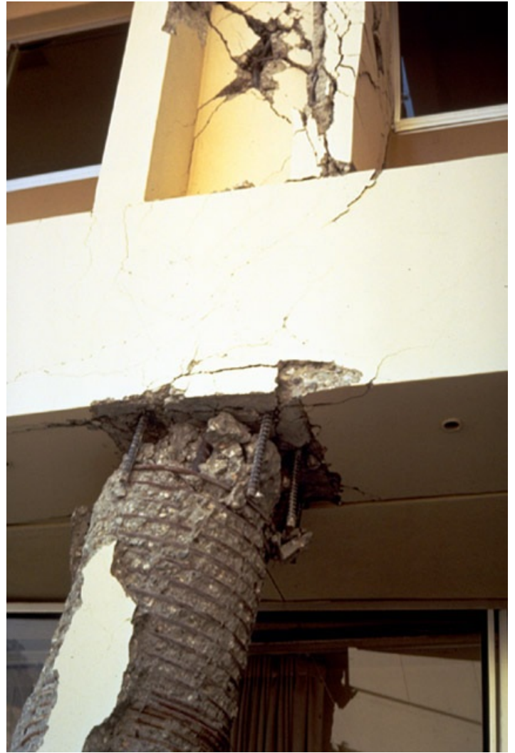
Olive View Hospital, 1971 San Fernando earthquake. Close-up of the top of the column illustrating how the concrete in this critical region has been disrupted (broken off) as a consequence of the premature ending of the spiral reinforcement. [10]
