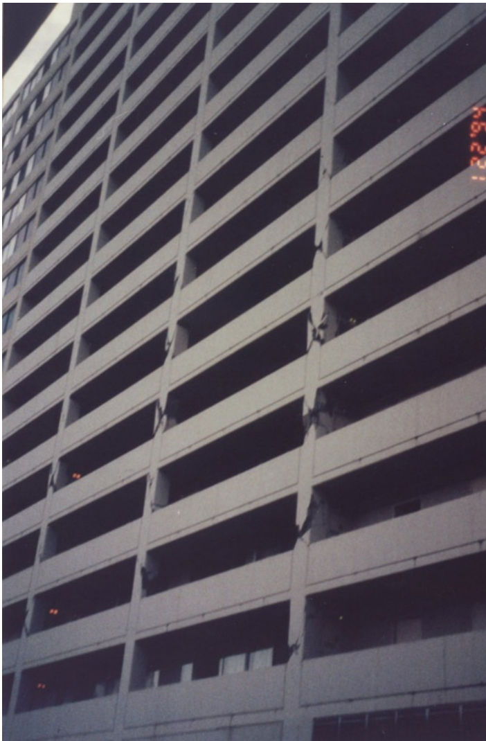
Damage from the 1994 Northridge earthquake to the perimeter moment frames of the Champaign Tower in Santa Monica, CA. [5]
