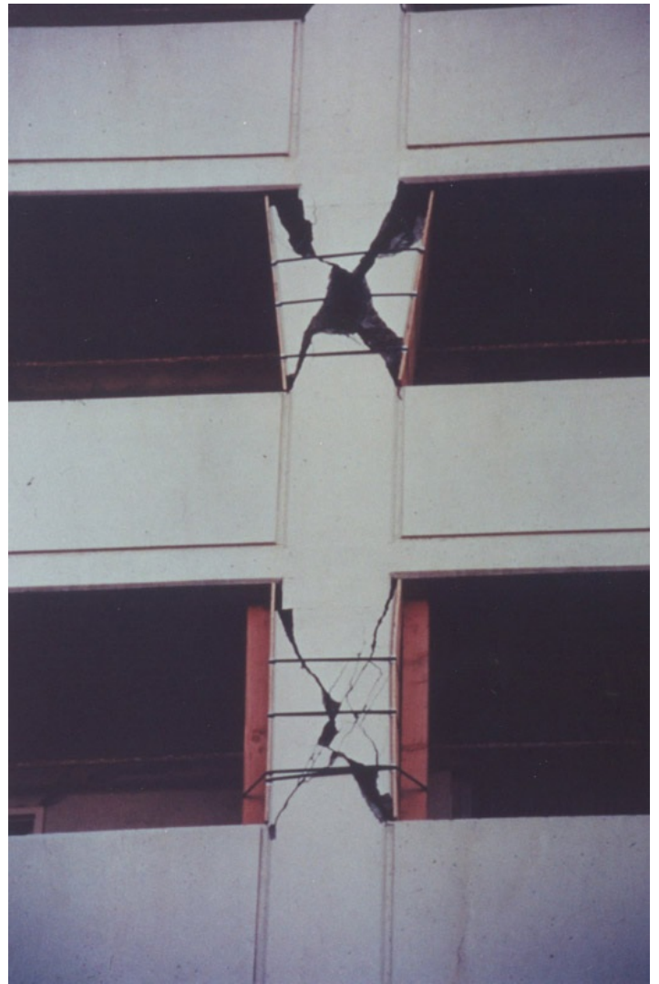
Balcony parapets induced short-column effects in the Champaign Tower moment frames. Typical X-shaped shear cracking from the short-column behavior is shown. [5]
