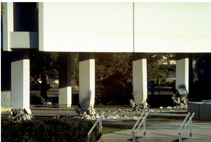
View of the 1979 Imperial Valley earthquake damage in the first story columns located in the east end of the Imperial County Services building. Note the explosive type of failure just above the ground.
