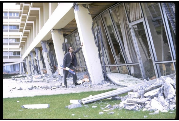
Damage to Olive View Hospital bottom story moment frame columns from the San Fernando earthquake. [9]
