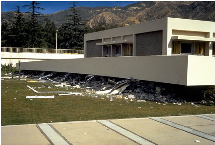
Olive View Hospital, Psychiatric Unit, 1971 San Fernando Earthquake. This unit was a 2-story reinforced concrete building. The structural system was a moment resisting frame.
