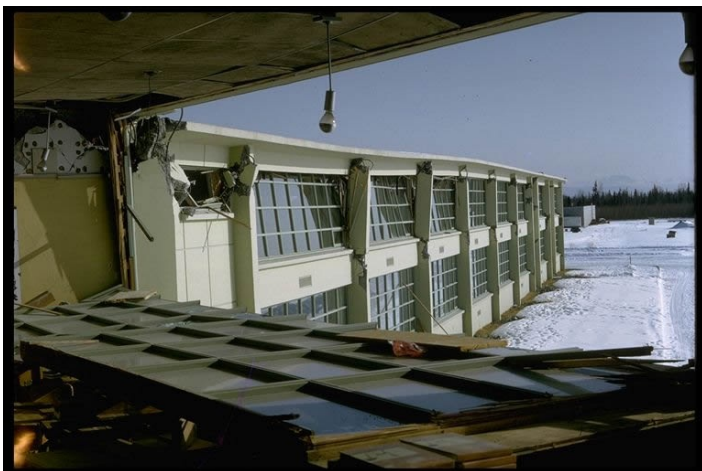
Damage to West Anchorage High School from the 1964 Alaska earthquake. Window wall fell inwards into the classrooms. Note sag in roof due to failure of
