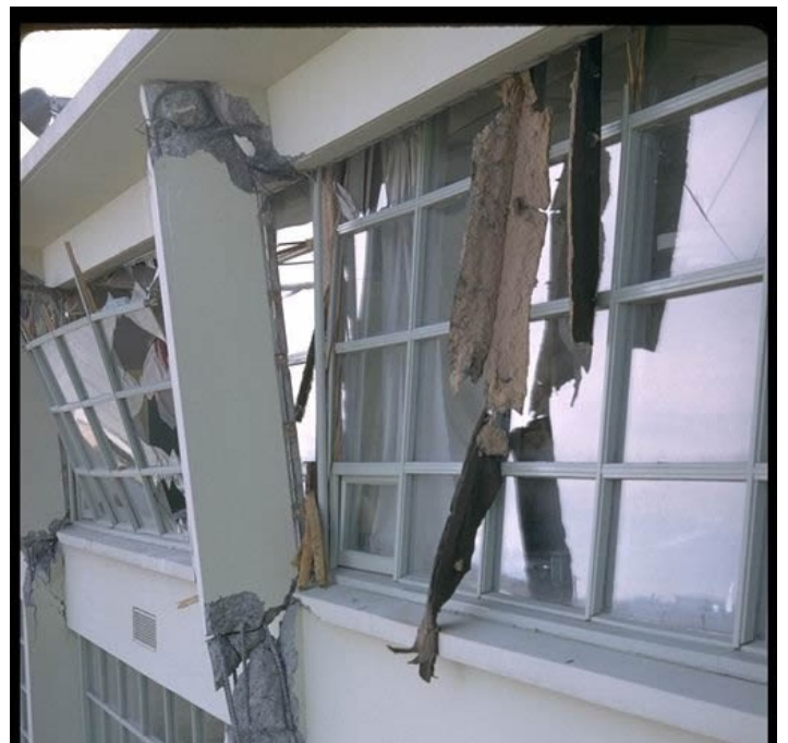
Close-up of characteristic X-shaped cracks and failure of coupling girders or short spandrel girders in the L street apartment building, Anchorage, Alaska. These girders were not properly designed for the shear demands. [10]
