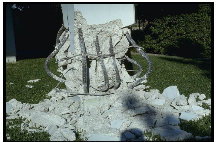
Close-up of the failure at the bottom of a column of the Imperial County Services building. The failure occurred in the zone of the column where there was not adequate confinement of the concrete and no
