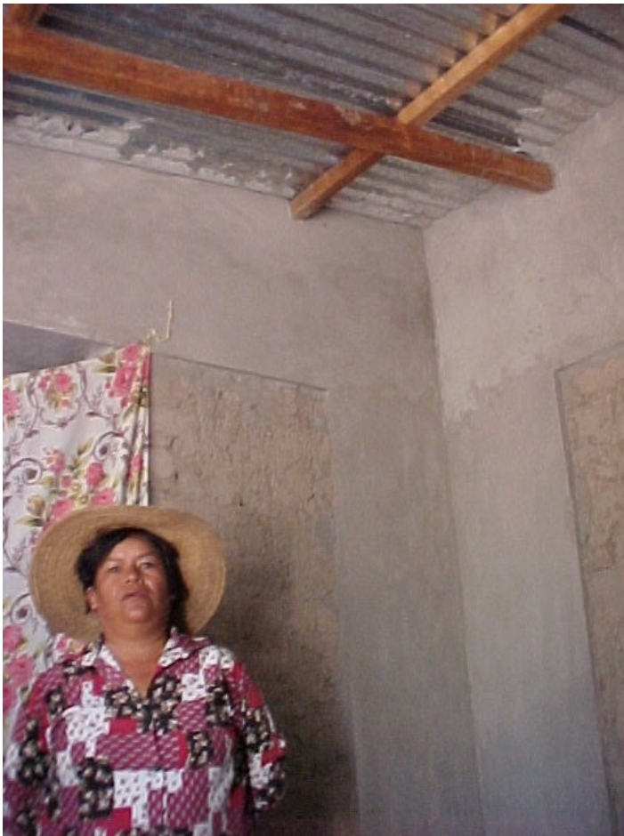
Interior wall strips and roof wood beams
