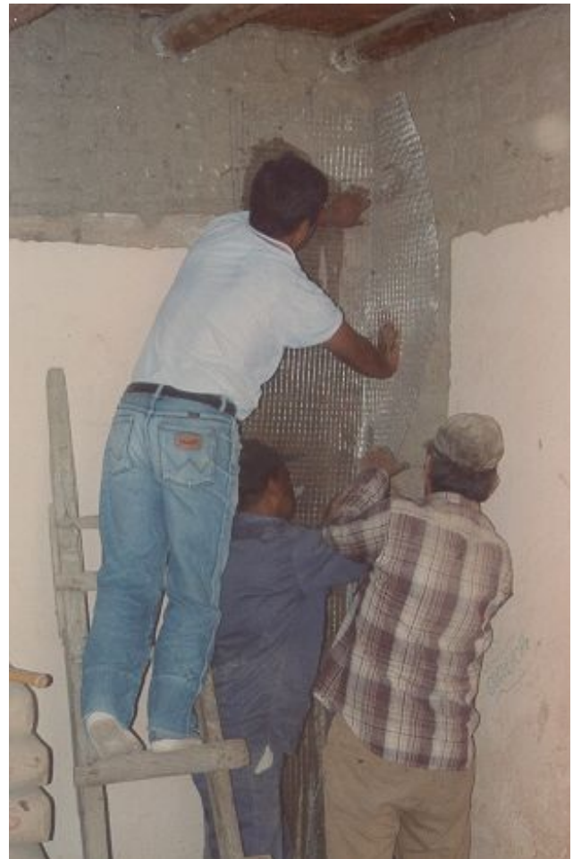
Placement of vertical strip of mesh at a corner
