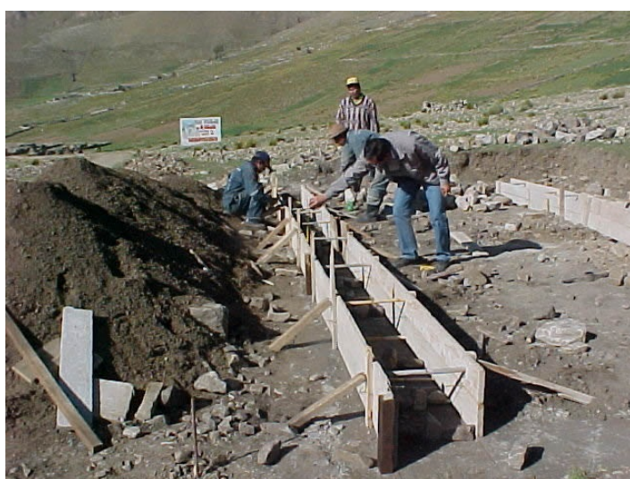
Plain concrete foundation
