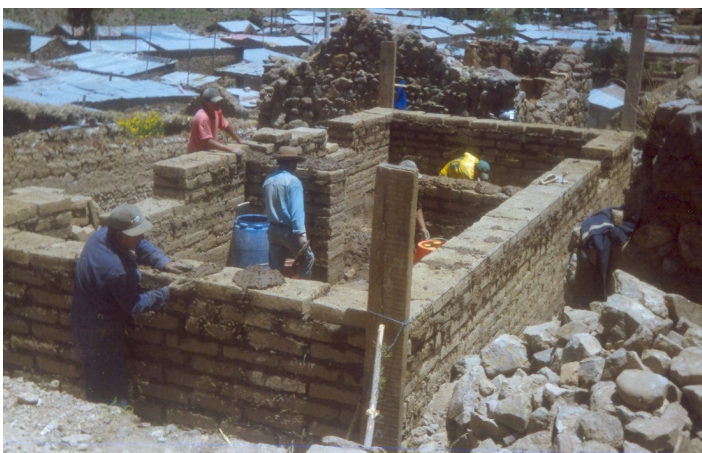
Adobe walls under construction
