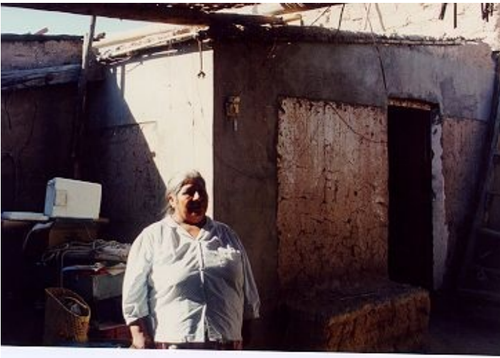
Adobe house reinforced with strips of wire mesh, undamaged after 2001 earthquake in Moquegua.
