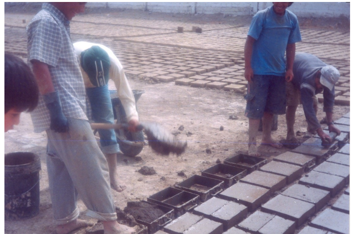
Adobe units under construction
