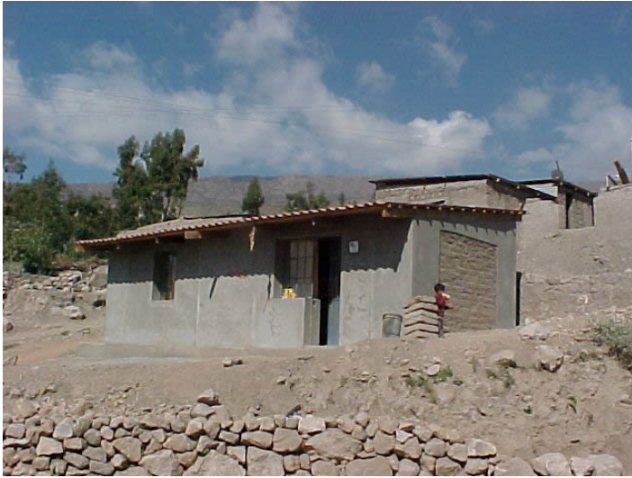
A typical rural street
