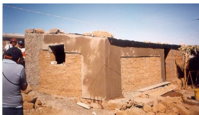
Bearing adobe walls are also the seismic resistant elements
