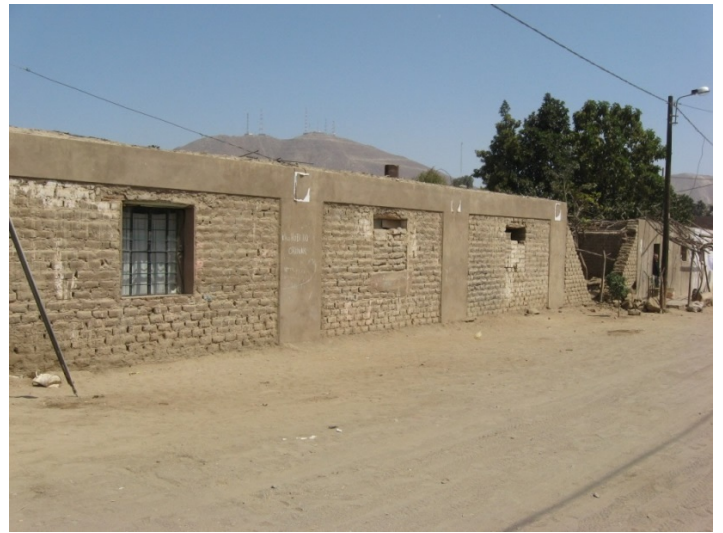
House in Ica after the 2007 earthquake, reinforced walls undamaged
