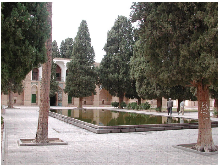
Historic adobe structure
