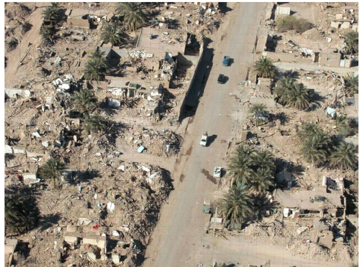
Aerial view of complete destruction of adobe dwellings in Bam earthquake
