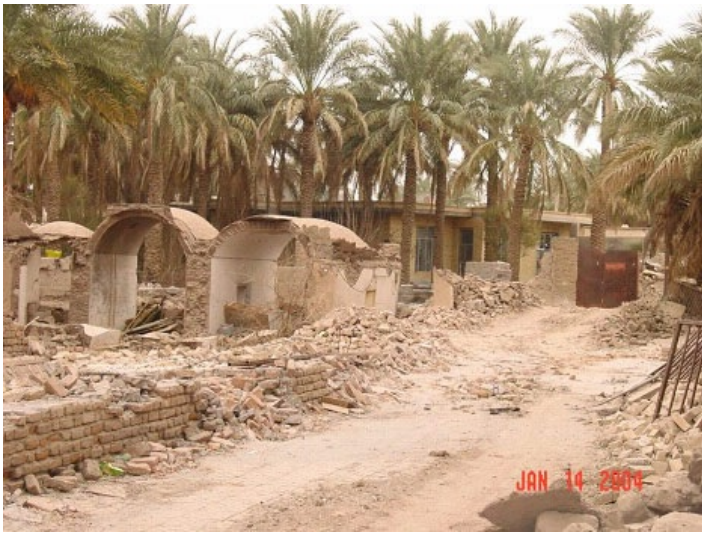
Key Seismic Deficiency--buildings not well-tied together. Example of building collapse in Bam earthquake
