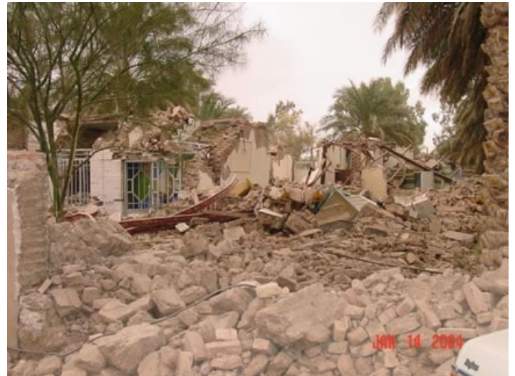
Bam earthquake: collapsed adobe structures
