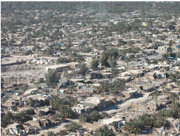
Aerial view of neighborhood with widespread damage to adobe
