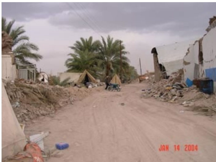
Bam earthquake: debris cleared from roadway, partially collapsed adobe structures, tents
