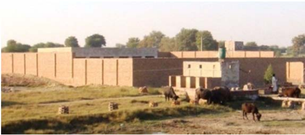
Figure 7. A relatively large brick house enclosed within a brick boundary wall, with detached outhouses.
