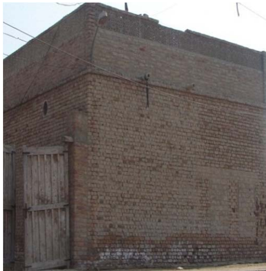
Figure 11. Brick masonry walls.
