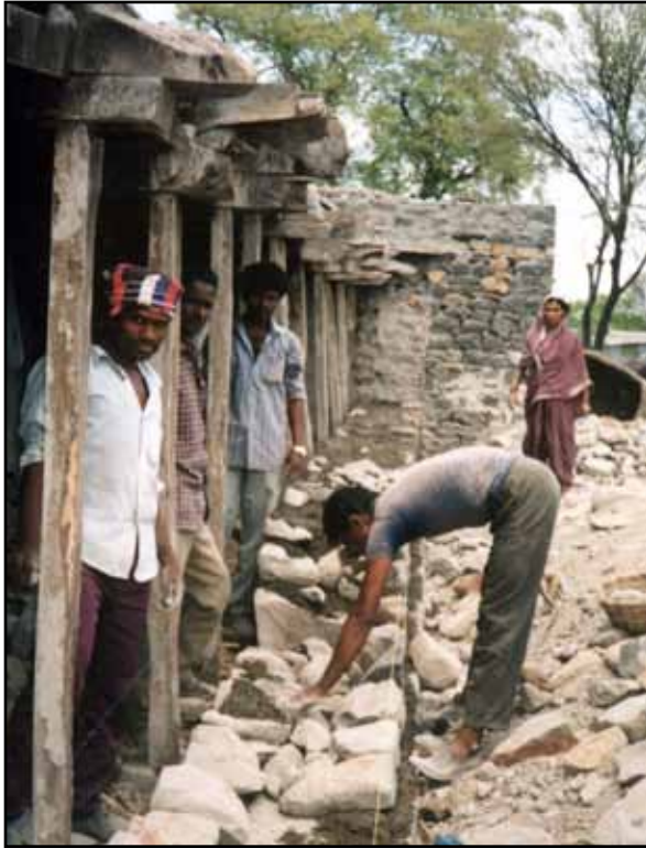
Figure 1.23 Construction of an uncoursed random rubble stone wall in Maharashtra, India (photo: S. Brzev)
