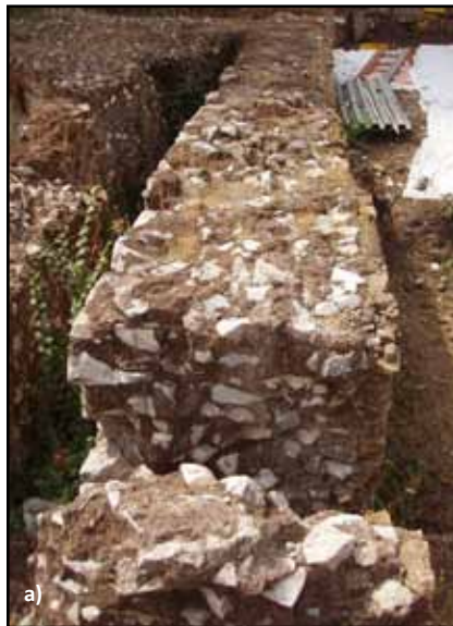
Figure 1.16 Concrete wall construction using stone rubble: a) an ancient Roman concrete wall, and b) in-situ concrete construction with stone rubble in Pakistan (photos: T. Schacher)
