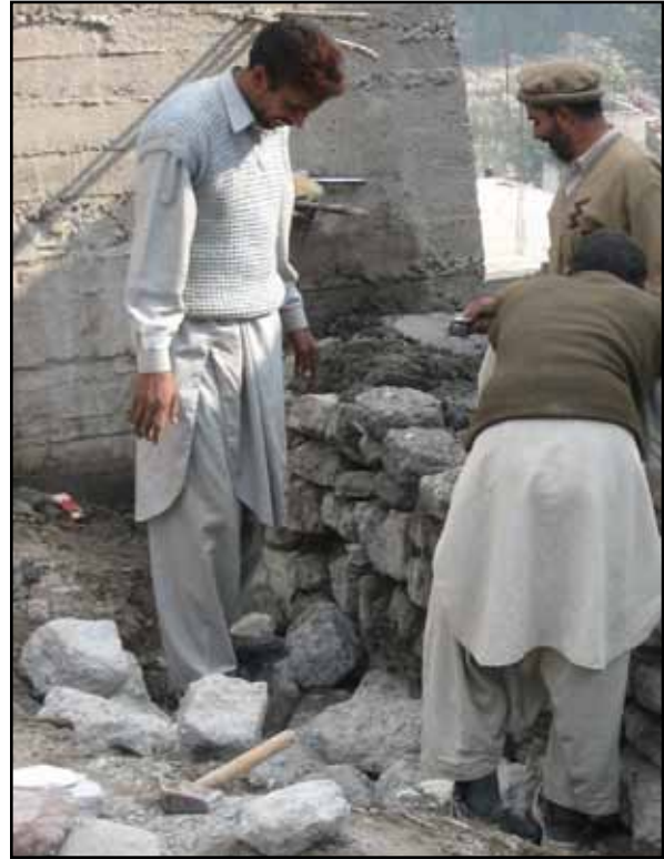
Figure 1.24 Construction of an uncoursed random rubble stone wall in Pakistan after the 2005 Kashmir earthquake (photo: M. Tomazevic)
