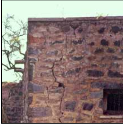
Figure 2.7 Vertical crack in a stone masonry wall due to the 1993 Maharashtra, India, earthquake (photo: S. Brzev)
