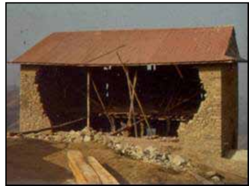
Figure 2.27 Out-of-plane collapse of a long wall in the 1988 East Nepal earthquake (photo: TAEC Consult, Nepal)
