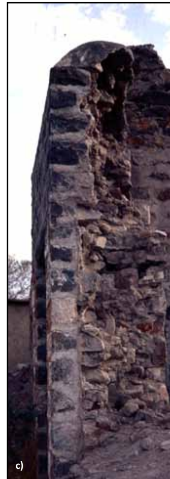
Figure 1.28 Stone masonry walls in Maharashtra, India: a) an uncoursed random rubble stone masonry wall (source: CBRI 1994); b) a semi-dressed stone wall with an exterior wythe built using wedge-shaped dressed stone (Source: CBRI, 1994), and c) an example of a semi-dressed stone wall (photo: S. Brzev)
