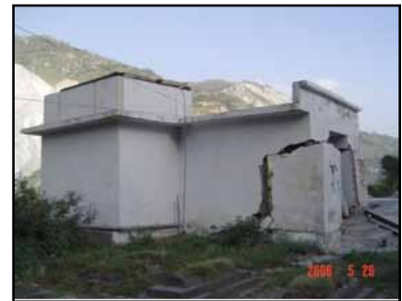
Figure 2.39 Soil spreading in the 2005 Kashmir, Pakistan, earthquake - note wide cracks in the walls (source: Bothara and Hıçyılmaz 2008)
