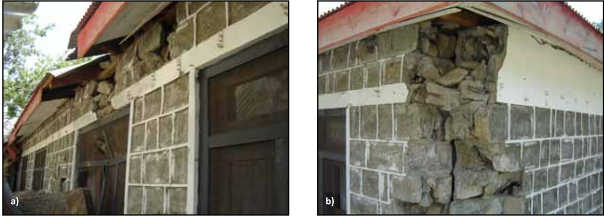
Figure 2.11 A stone masonry building with an RC lintel band that survived the 2005 Kashmir earthquake in Pakistan: a) the building suffered only moderate damage in the top portion, and b) separation at the wall intersection took place in spite of the band (note inadequate anchorage of the band reinforcement) (photos: Builders Without Borders)
