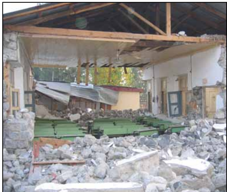
Figure 2.27 Out-of-plane collapse of a long wall in the 1988 East Nepal earthquake (photo: TAEC Consult, Nepal)
