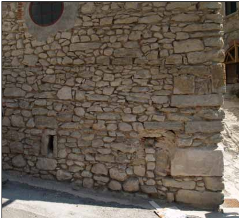
Figure 1.25 A building with uncoursed stone masonry walls in lime mortar in L'Aquila, Italy (note round stone boulders) (photo: T. Schacher)
