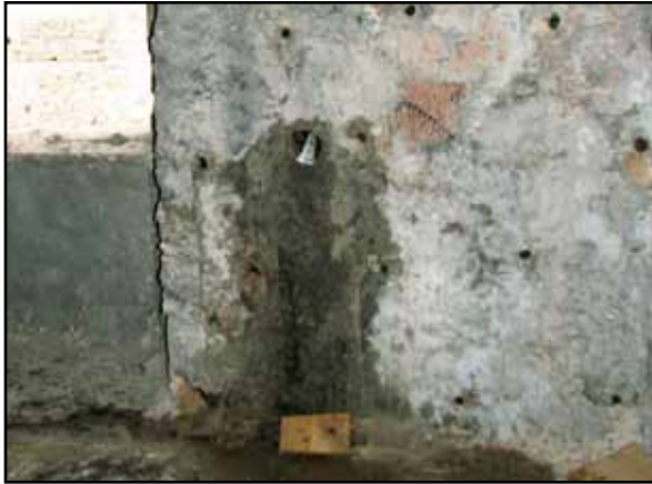
Figure 4.27 Grouting an existing stone masonry wall in Slovenia - note uniformly distributed holes at the location where grout is to be injected (photo: M. Lutman)
