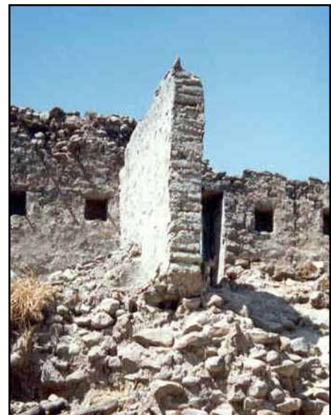
Figure 1.18 A wall without foundations in the area affected by the 1993 Maharashtra, India, earthquake (photo: S. Brzev)
