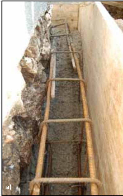
Figure 4.30 Strengthening a stone masonry foundation: a) reinforcement cage and formwork, and b) new reinforced concrete foundation under construction (photos: M. Lutman)
