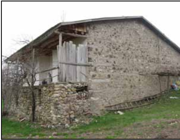
Figures 1.3 Typical stone masonry houses in Turkey (photos: M. Erberik)
