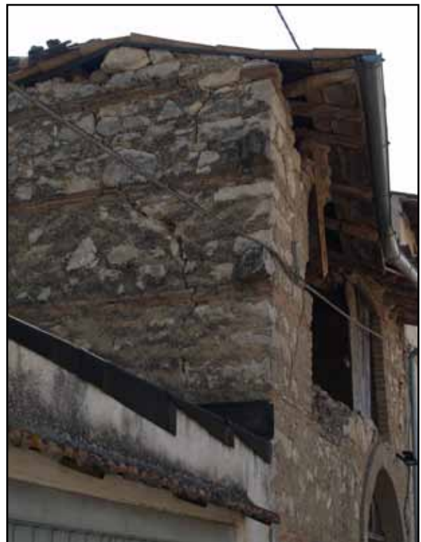
Figure 1.30 A stone masonry wall with brick bands in L'Aquila, Italy (photo: T. Schacher)
