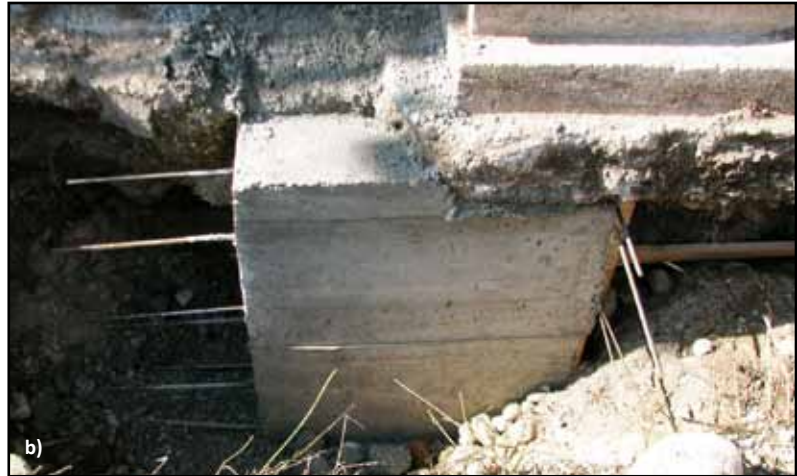
Figure 4.30 Strengthening a stone masonry foundation: a) reinforcement cage and formwork, and b) new reinforced concrete foundation under construction (photos: M. Lutman)
