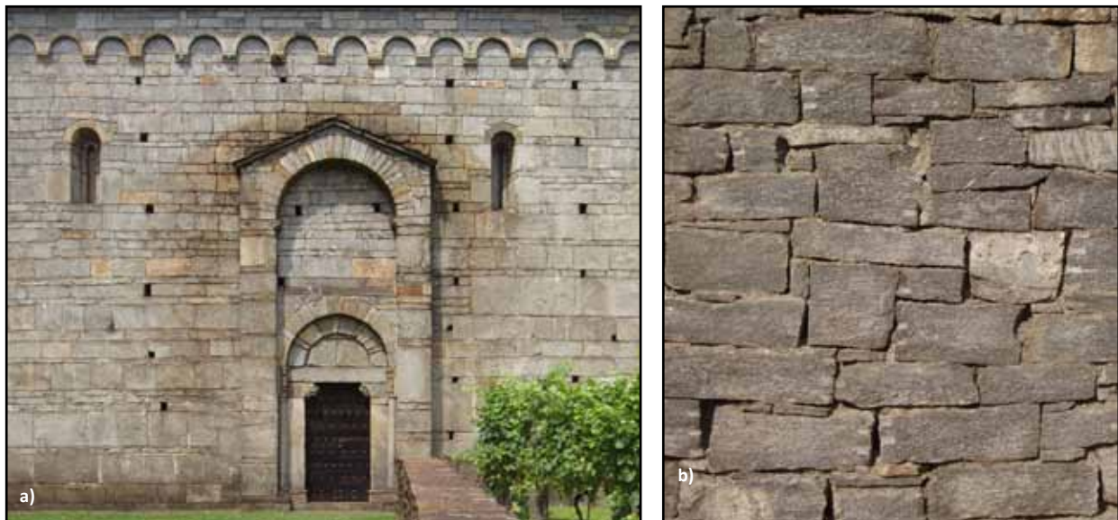
Figure 1.32 Dressed stone masonry construction in Southern Switzerland: a) a typical building in Giornico, and b) a detail of the exterior (photos: T. Schacher)
