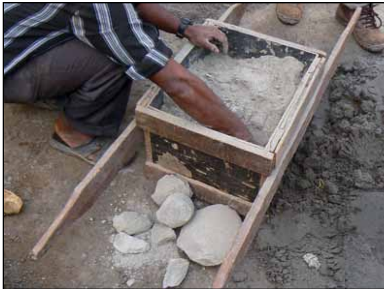
Figure 3.43 Cement with large lumps should not be used for construction (photo: Smart Shelter Foundation)
