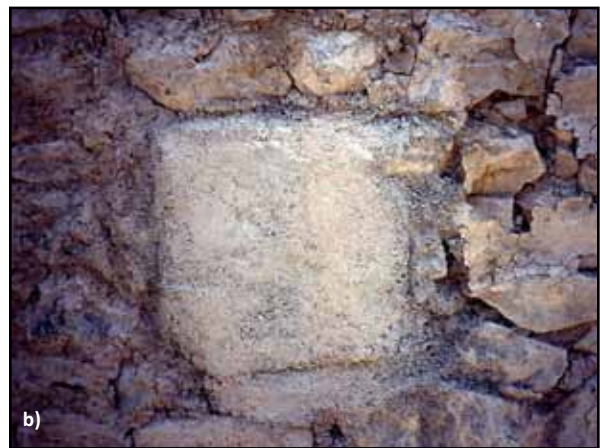
Figure 4.19 Examples of through-stone installation in Maharashtra, India: a) removing stone from the existing wall, and b) surface of a through-stone covered with a plaster (photos: S. Brzev)
