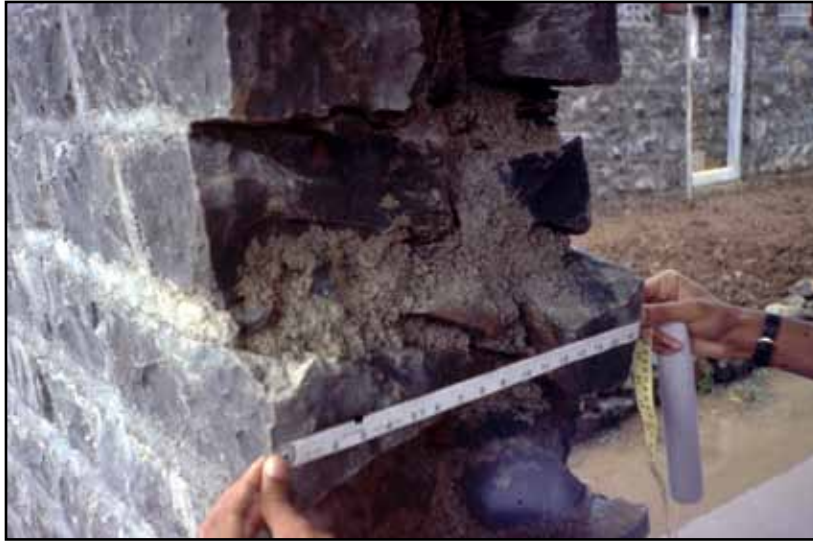
Figure 3.27 Examples of stone masonry in cement mortar with a wall thickness limited to 450 mm (note through-stones) (photos: S. Brzev)
