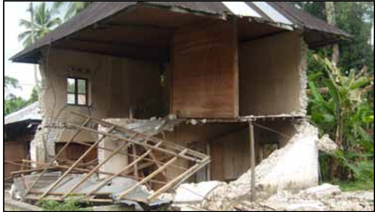
Figure 2.29 (left and above) Out-of-plane collapse of stone masonry walls in the 2009 Padang, Indonesia, earthquake (source: Bothara et al. 2010)
