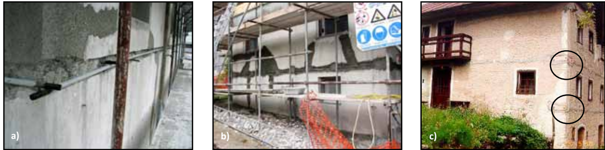
Figure 4.4 A field application of ties in Slovenia: a) and b) installation of steel ties after the 1998 Bovec, Slovenia, earthquake (note that anchorage end-plates are yet to be attached), and c) an example of a retrofitted building (photos: M. Lutman)
