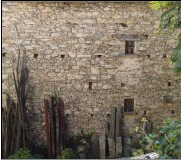
Figure 1.26 Uncoursed semi-dressed stone masonry wall in Southwestern Switzerland (photo: T. Schacher)
