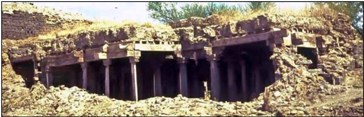
Figure 2.19 Wall collapse in the 1993 Maharashtra, India, earthquake: a stone masonry building with a timber roof and a heavy mud overlay (photo: S. Brzev)
