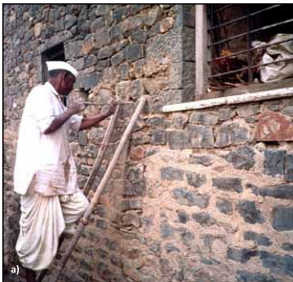
Figure 4.19 Examples of through-stone installation in Maharashtra, India: a) removing stone from the existing wall, and b) surface of a through-stone covered with a plaster (photos: S. Brzev)
