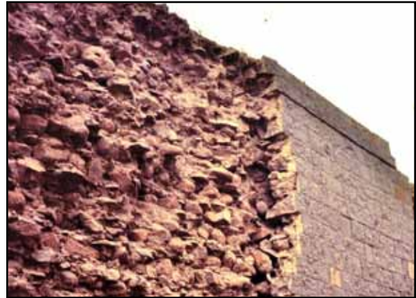
Figure 2.23 Delamination was a common damage pattern observed in the 1993 Maharashtra, India, earthquake (photos: S. Brzev)
