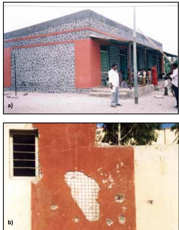
Figure 4.11 Strengthening of intersecting walls: a) retrofitted school building in India, and b) an unsuccessful retrofit application (photos: S. Brzev)
