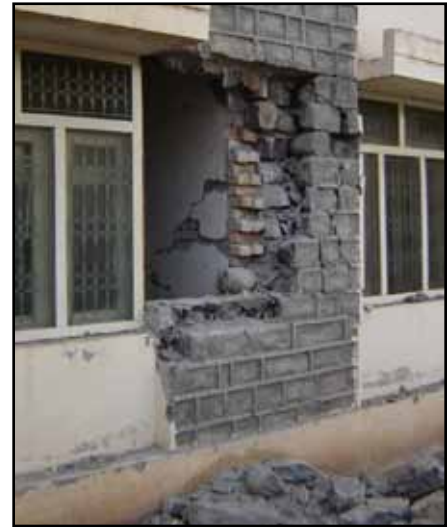
Figure 2.38 Vertical cracking at a wall intersection in the 2005 Kashmir, Pakistan, earthquake due to absence of connection between the intersecting walls, a stone masonry and a brick-masonry wall (source: Bothara and Hıçyılmaz 2008)
