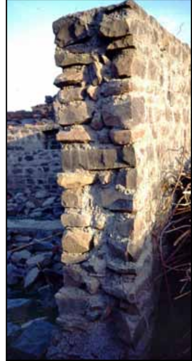
Figure 3.27 Examples of stone masonry in cement mortar with a wall thickness limited to 450 mm (note through-stones) (photos: S. Brzev)
