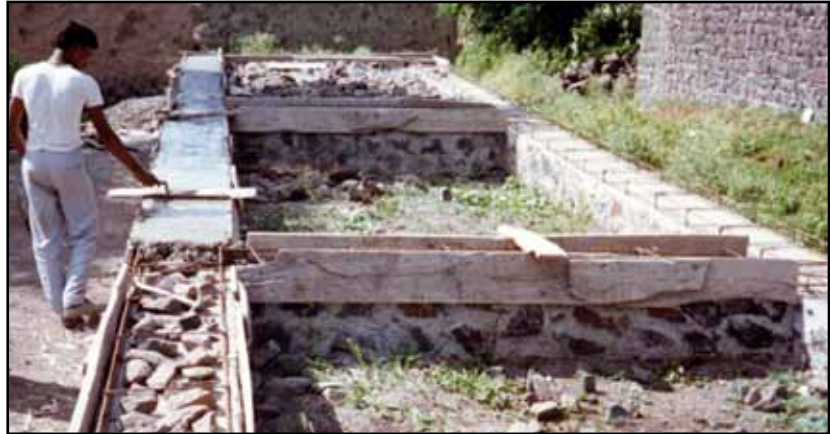
Figure 3.39 Construction of an RC plinth band using large stone rubble (also known as "stone-crete") (photo: S. Brzev)
