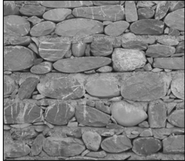
Figure 1.27 Stone masonry wall built using round river stone boulders with shaped exterior surfaces near Balakot, Pakistan (photo: T. Schacher)
