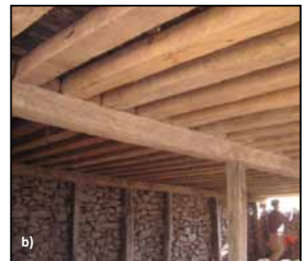
Figure 1.7 Dual gravity load-bearing system: a) a typical stone masonry building with exterior stone masonry walls and an interior timber frame in Maharashtra, India (source: GOM 1998), and b) a stone masonry building with dual system under construction in Pakistan (source: Bothara and Hıçyılmaz 2008)
