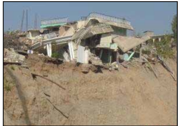
Figure 3.3 A building damaged by a landslide in the 2005 Kashmir, Pakistan, earthquake (source: Bothara and Hıçılmaz 2008)
