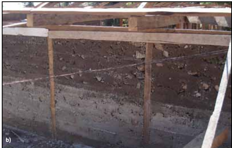
Figure 1.16 Concrete wall construction using stone rubble: a) an ancient Roman concrete wall, and b) in-situ concrete construction with stone rubble in Pakistan (photos: T. Schacher)
