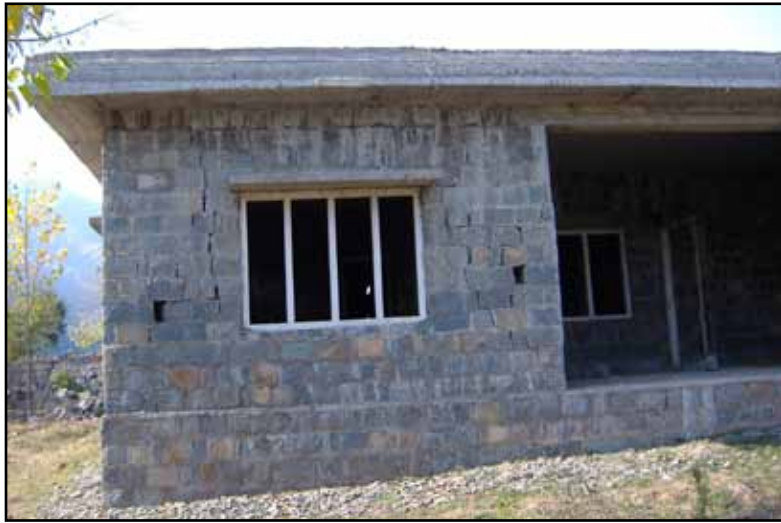
Figure 1.14 A stone masonry building with an RC slab roof in Pakistan (photo: J. Bothara)
