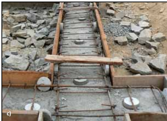
Figure 3.19 Concrete cover in RC bands: a) exposed bars due to inadequate cover, b) concrete spacers made from PVC pipes, and c) RC band under construction showing use of concrete spacers (photos: Smart Shelter Foundation)
