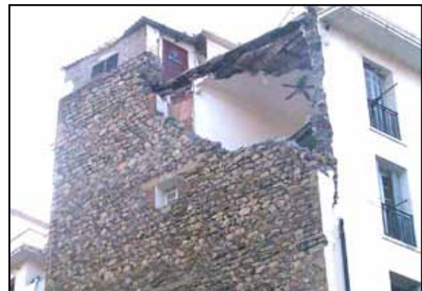
Figure 2.25 Out-of-plane collapse at the top floor of a stone masonry building in the 2003 Boumerdes earthquake in Algeria (photo: M. Farsi)
