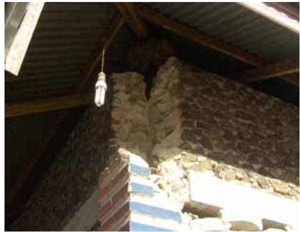
Figure 2.9 Damage at a wall intersection of a single-story stone masonry building in the 2009 Padang, Indonesia, earthquake (note absence of bands at lintel and roof levels) (source: Bothara et al. 2010)
