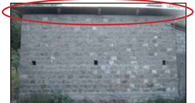
Figure 2.10 A stone masonry building in Muzaffarabad was undamaged in the 2005 Kashmir, Pakistan, earthquake; this was attributed to the presence of an RC band at the eaves level (photo: J. Bothara)
