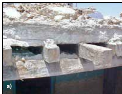
Figure 2.14 Roof deficiencies in the area affected by the 2001 Bhuj, India, earthquake: a) discontinuous rafters over interior walls, and b) inadequate wall-to-floor connections caused the severe building damage (photos: C.V.R. Murty)
