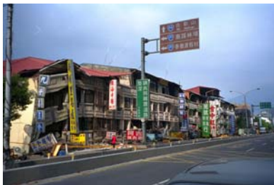
Figure 6D: Earthquake Damage - Pancake Collapse of an Entire City Block in the 1999 Chi Chi earthquake (Source: EERI 2001)
