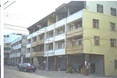
Figure 1B: Typical Building (Source: EERI 2001)
