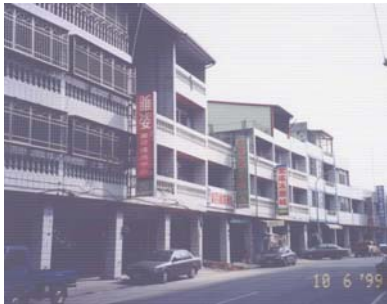
Figure 1A: Typical Building
