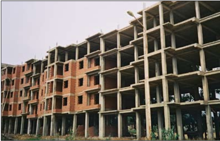
Figure 3: RC frame construction with hollow-clay tile masonry infill in Algeria (Credit: S. Brzev)
