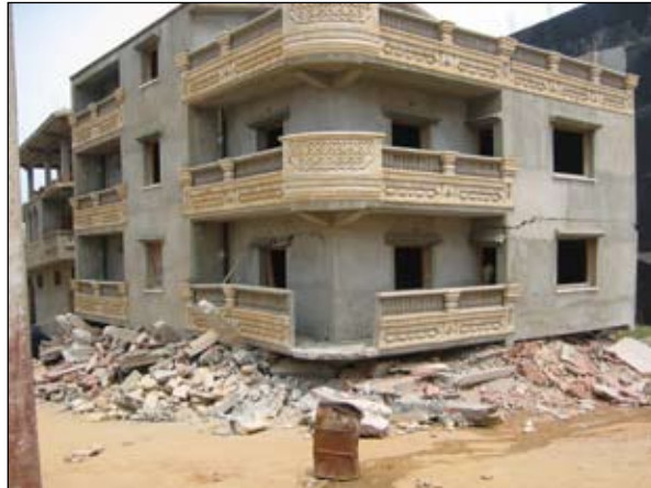
Figure 7: Building collapse due to soft-story mechanism in the 2003 Boumerdes earthquake (WHE Report 103, Algeria)
