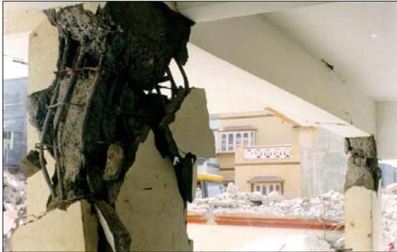
Figure 5: Shear failure of a reinforced concrete column in the 2001 Bhuj earthquake (WHE Report 19, India)
